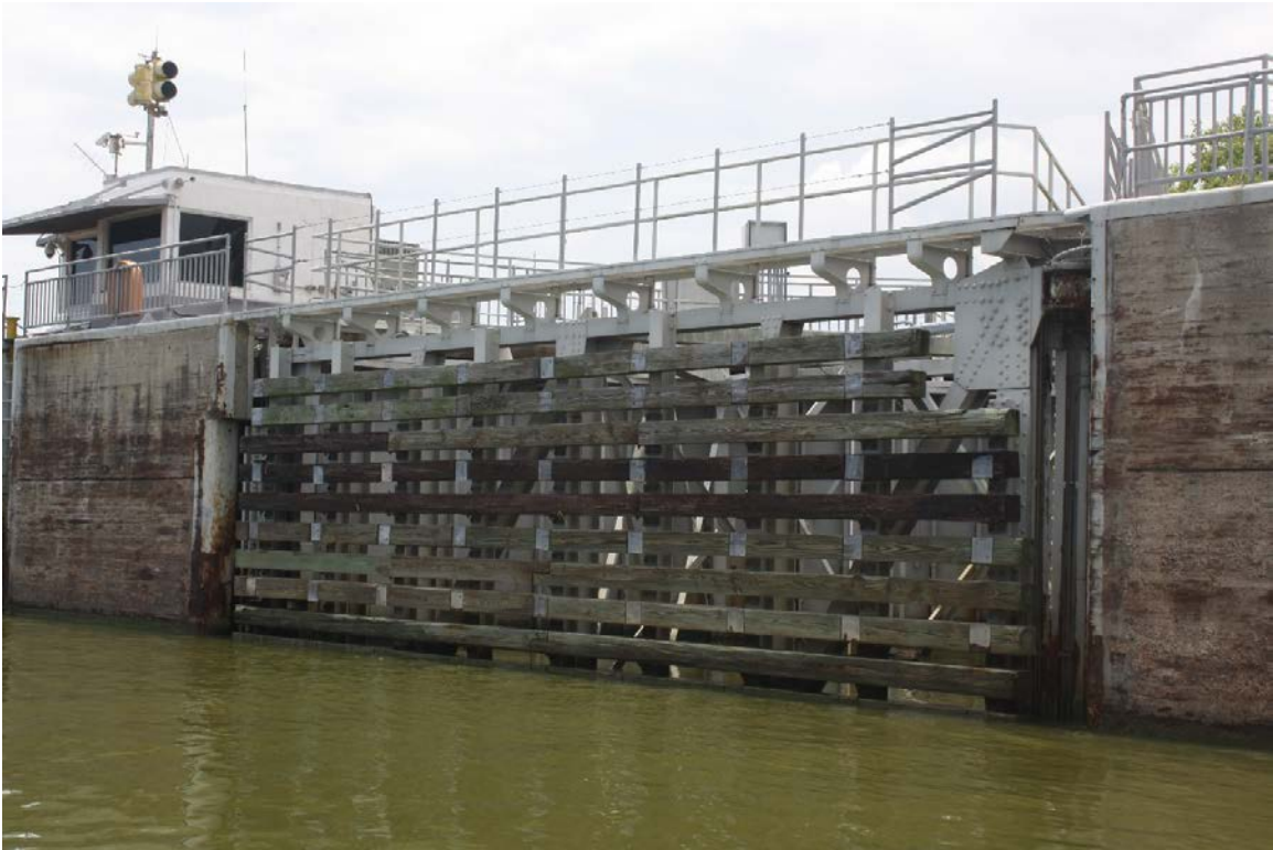
View of north 1944 lock gate, facing west
