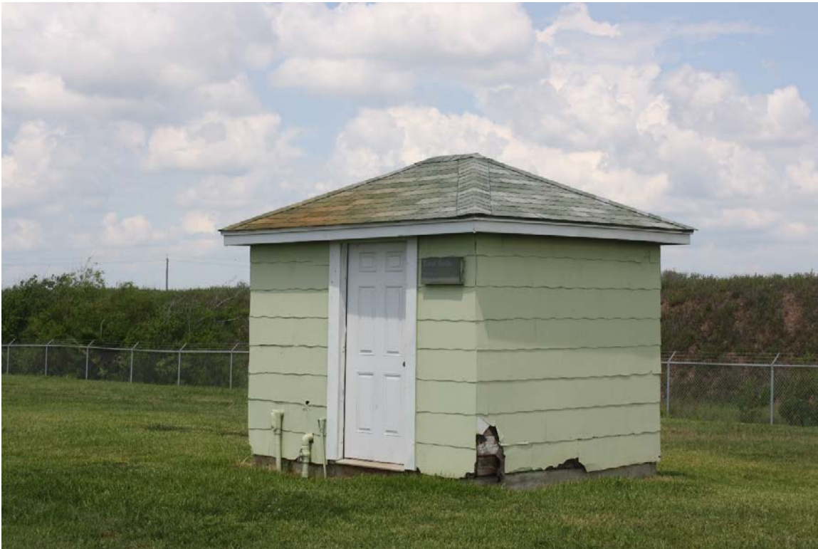
Oblique view of pumphouse, facing west
