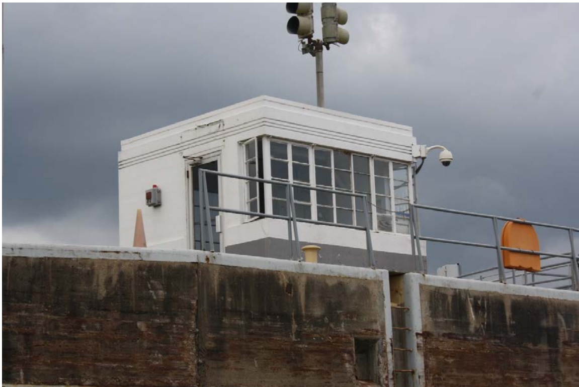
View of 1951 control house, facing north
