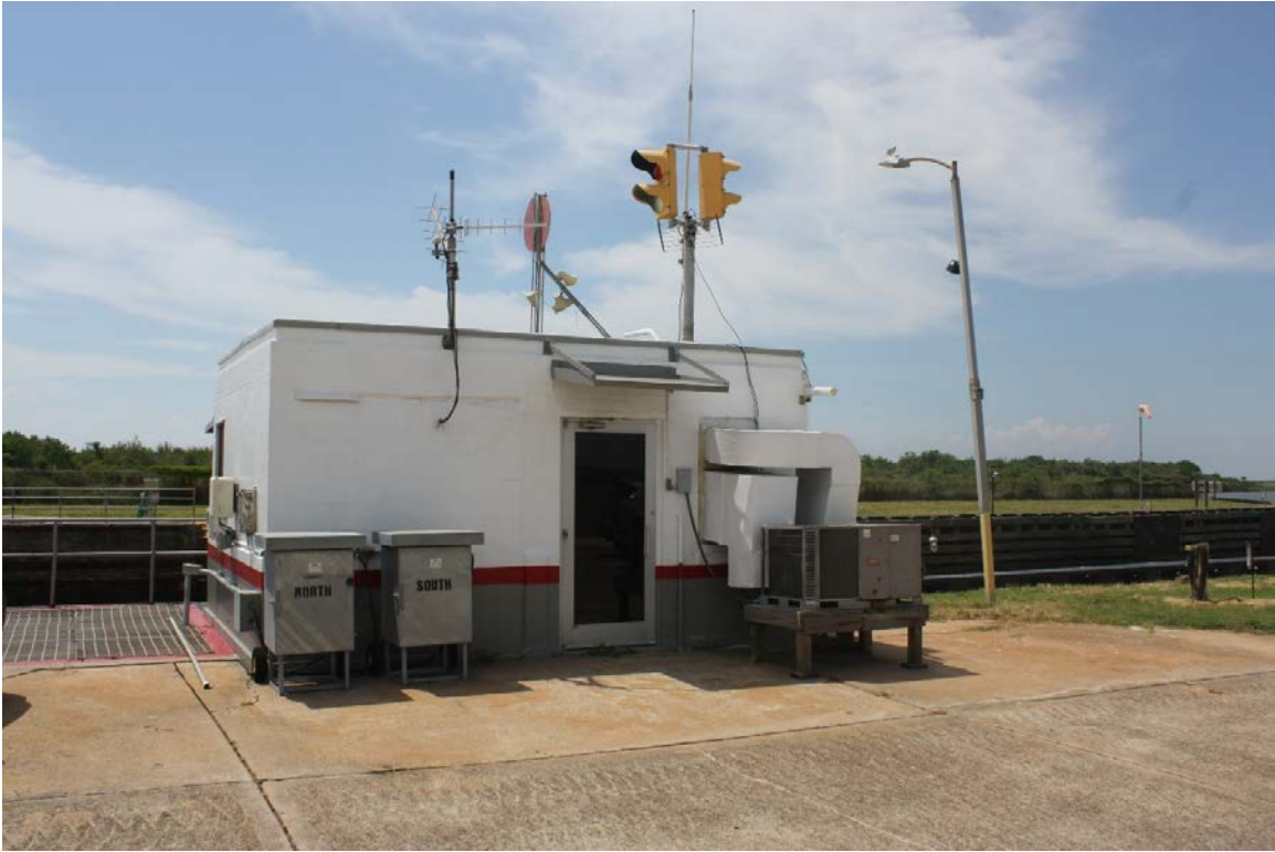
View of north elevation, facing south
