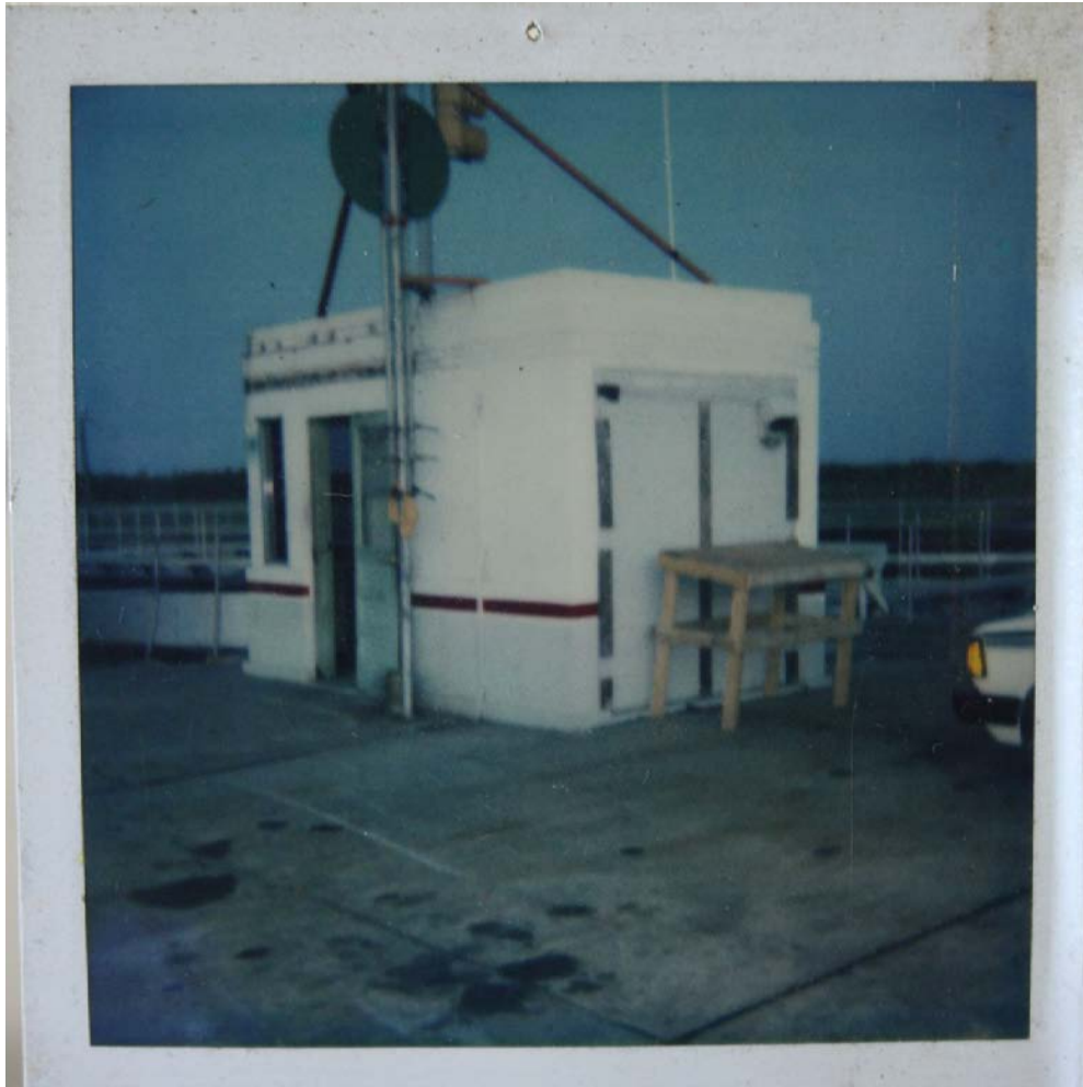
Photo dated to the 1970s showing the original size and Moderne detailing of the west control house. The multi-light windows have been replaced. Image courtesy USACE.
