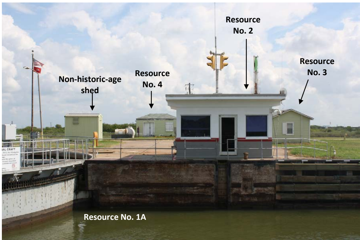
D6: View showing relationship of west floodgate, control house, power house, and restroom/shed, facing northeast from GIWW
