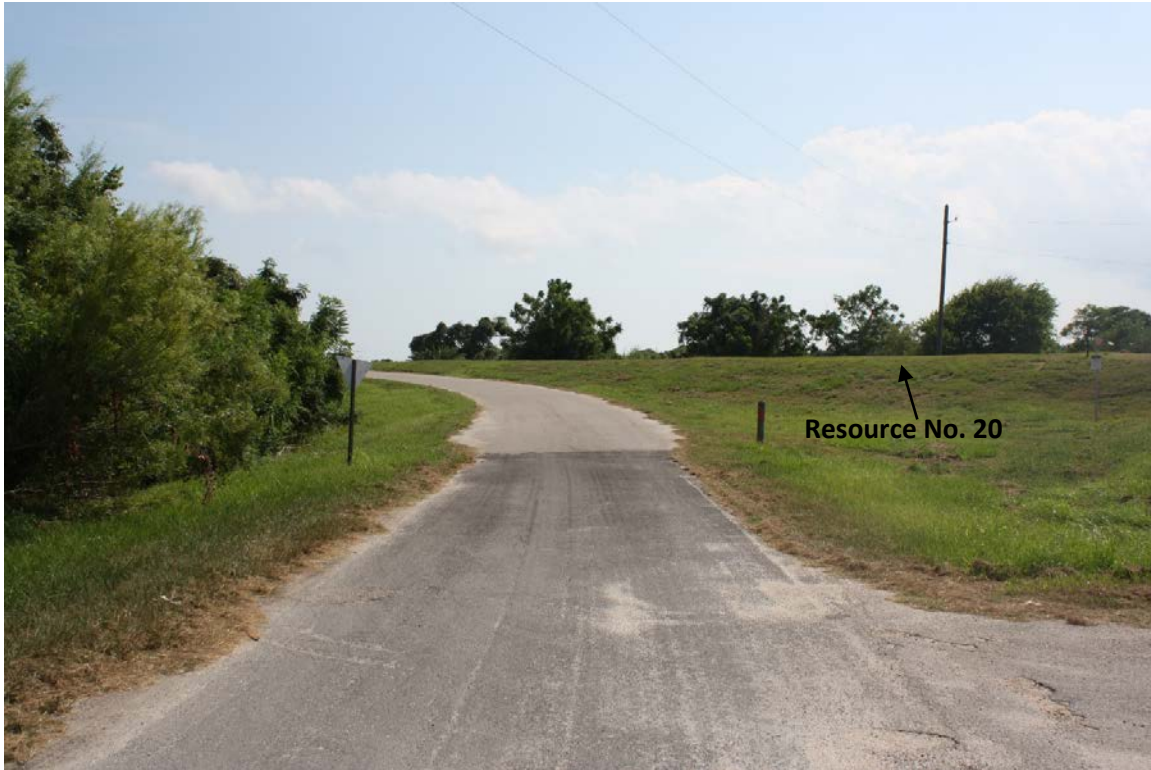
D23: View of levee (Resource No. 20) and west lock access road, facing southwest from Matagorda Ave
