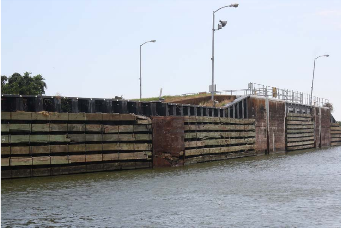
Representative photo of damage to timber fenders and steel sheets, facing south
