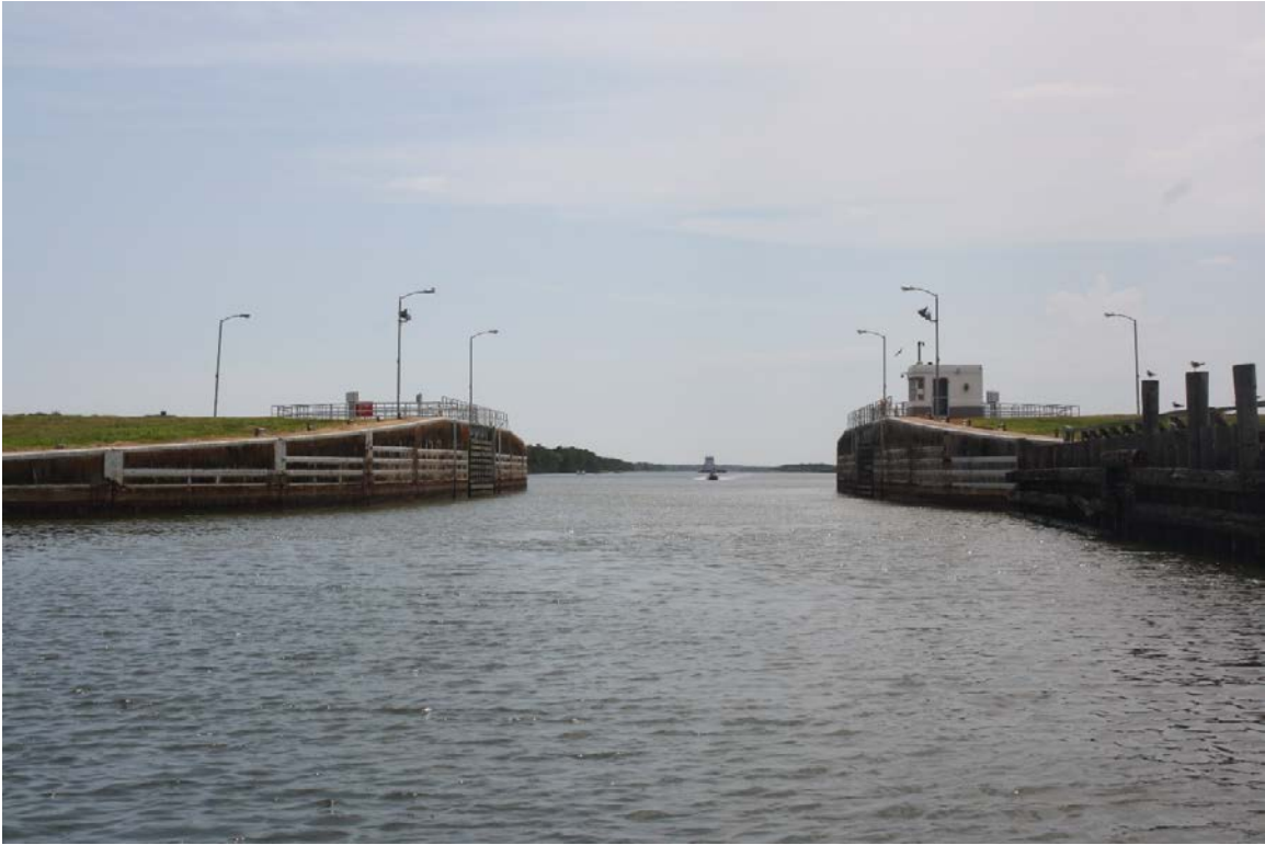
View of 1951 lock gates, facing southwest
