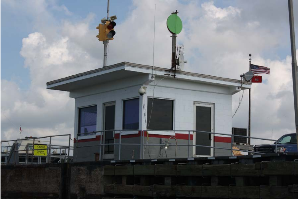
View of Brazos River west floodgate control house, facing northwest
