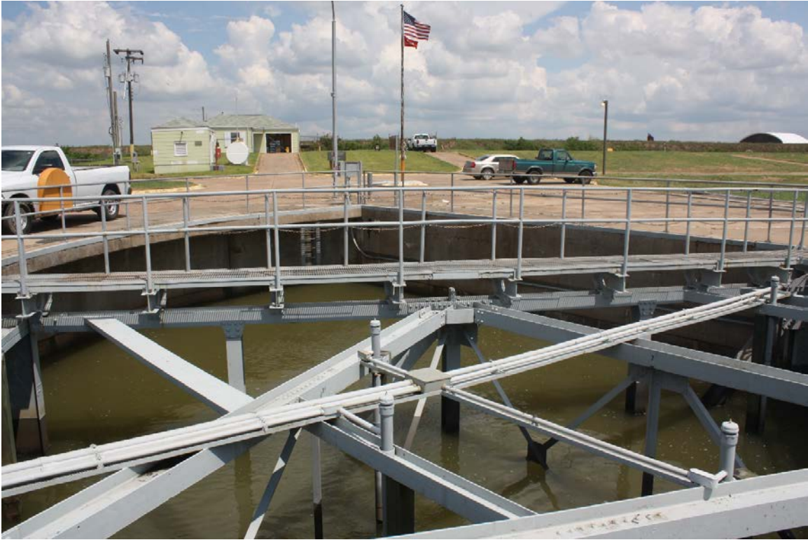
View of representative concrete recess well, facing north
