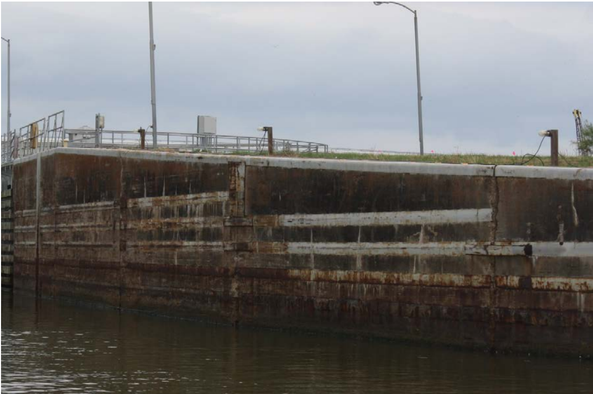
Representative view of cracking concrete and steel corrosion, facing east
