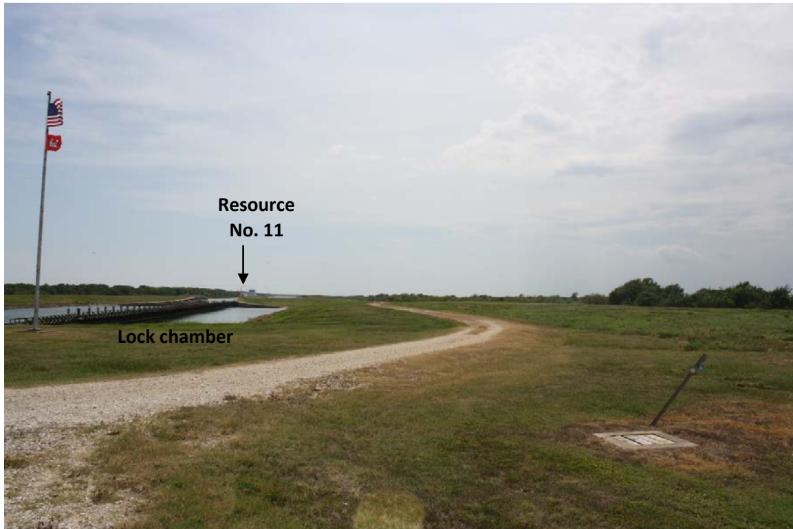
D17: View of internal access road from 1944 control house (Resource No. 12), facing southwest
