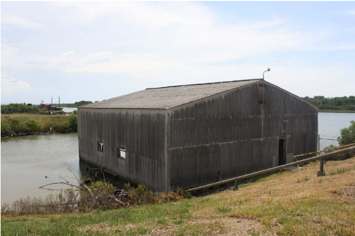
Oblique view, facing east from internal access road
