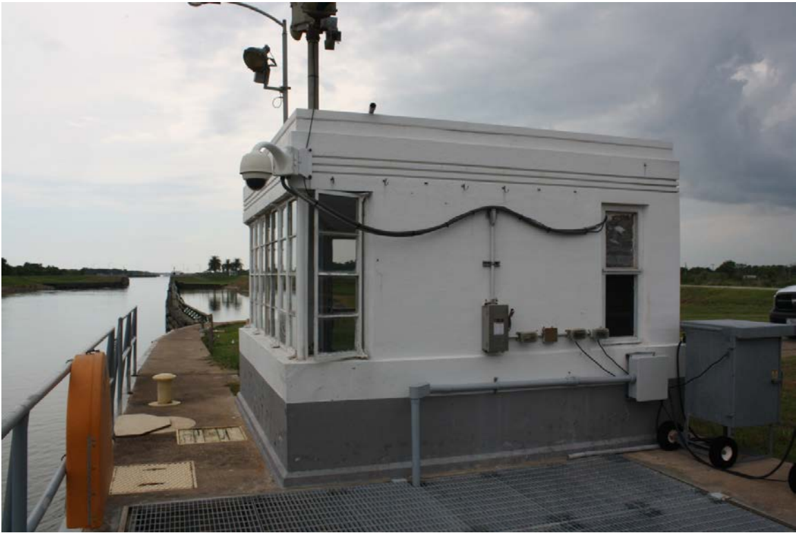
View of east elevation, facing southwest
