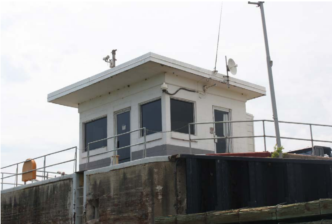
View of control house, facing west
