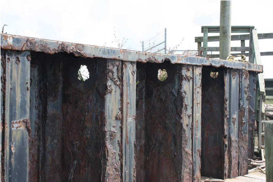
Representative view of section loss, pack rust, and corrosion in steel section of guide wall, facing north
