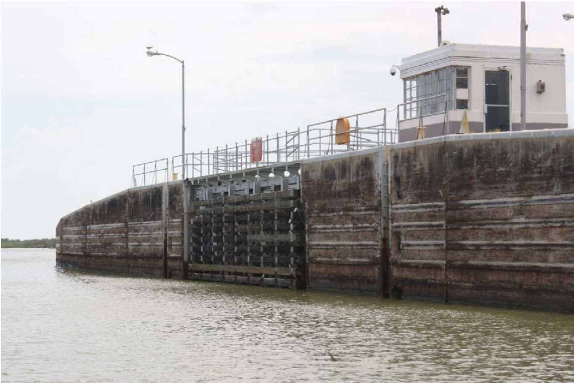
View of 1951 north lock gate and control house, facing west
