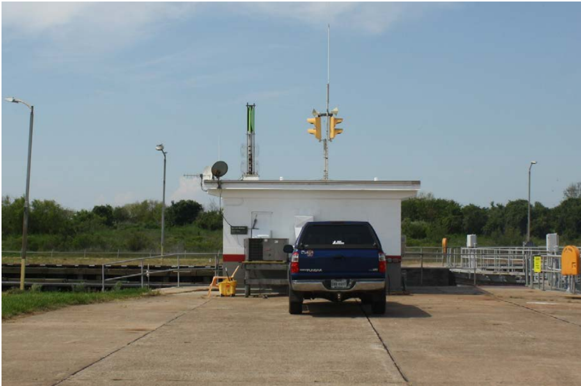
View of rear (north) elevation of control house, facing southwest
