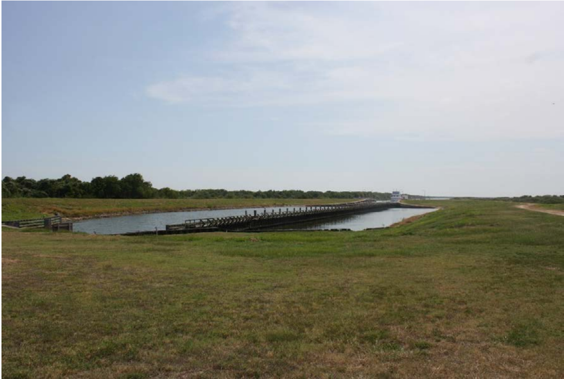
View of lock chamber from 1944 control house (Resource No. 12), facing southwest
