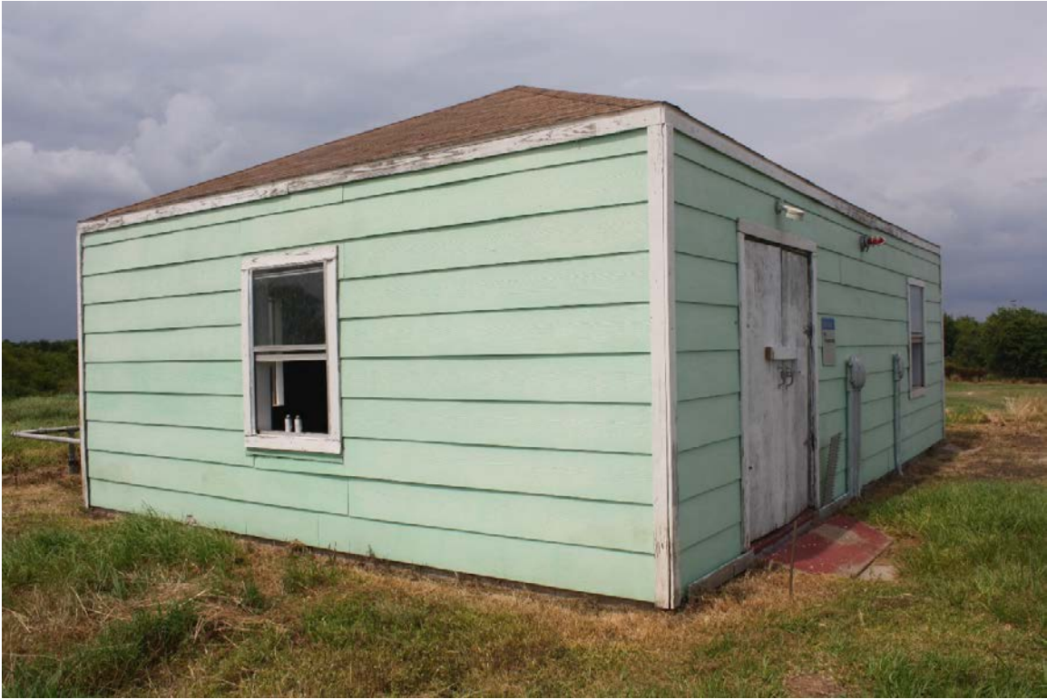
Oblique view of power house, facing north
