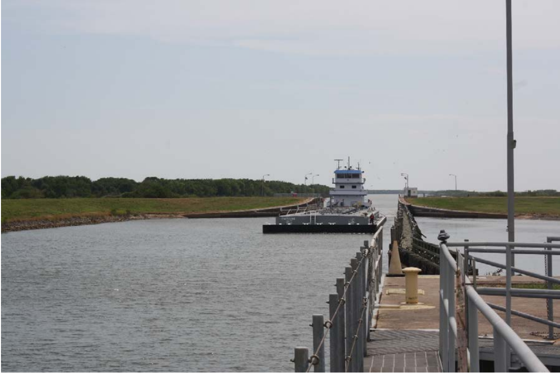
D21: Barge traveling east through west lock, facing southwest toward 1951 control house (Resource No. 11)
