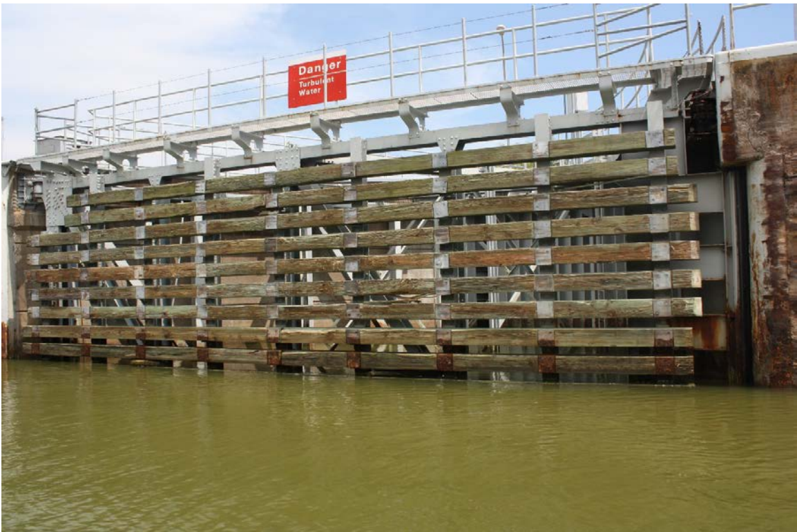
View of 1951 south lock gate, facing west
