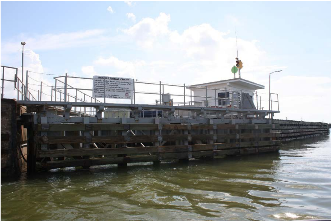
Representative view of gate in process of opening, facing northeast. Control house (Resource No. 2) is in the background.
