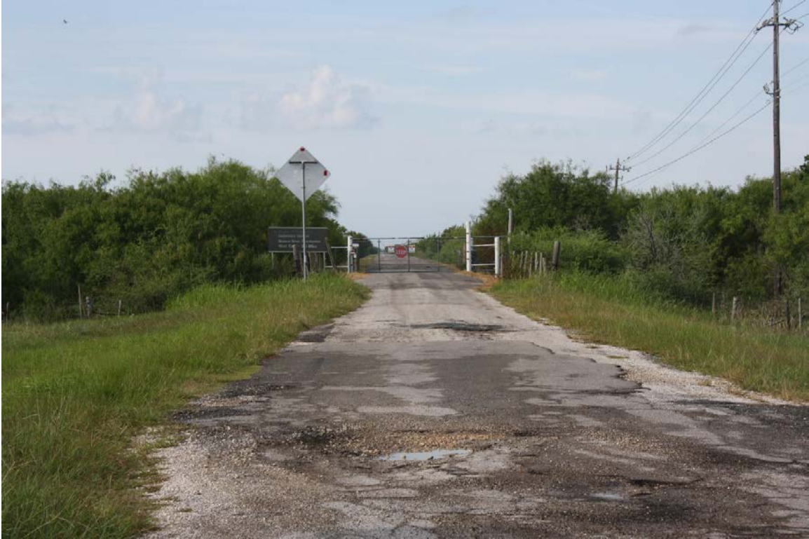
D1: View of west floodgate access road from SH 36, facing southwest. Access road is 3.5 miles in length.
