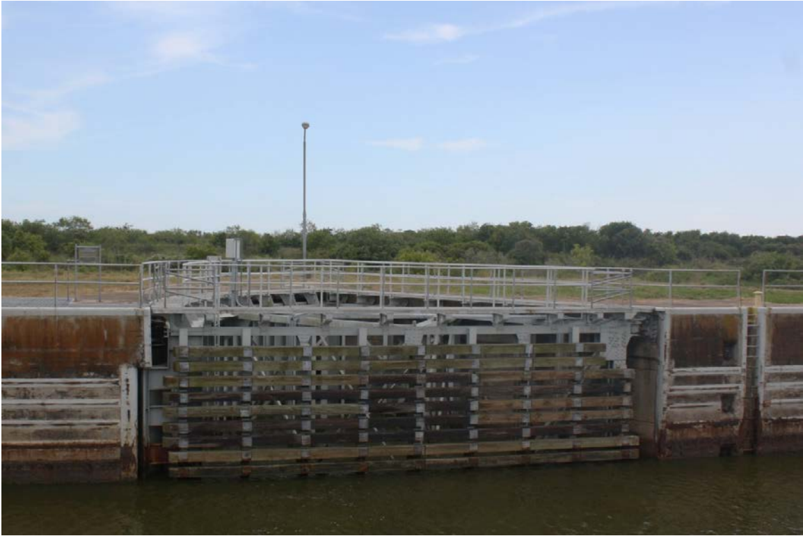
View of 1951 south lock gate, facing southwest
