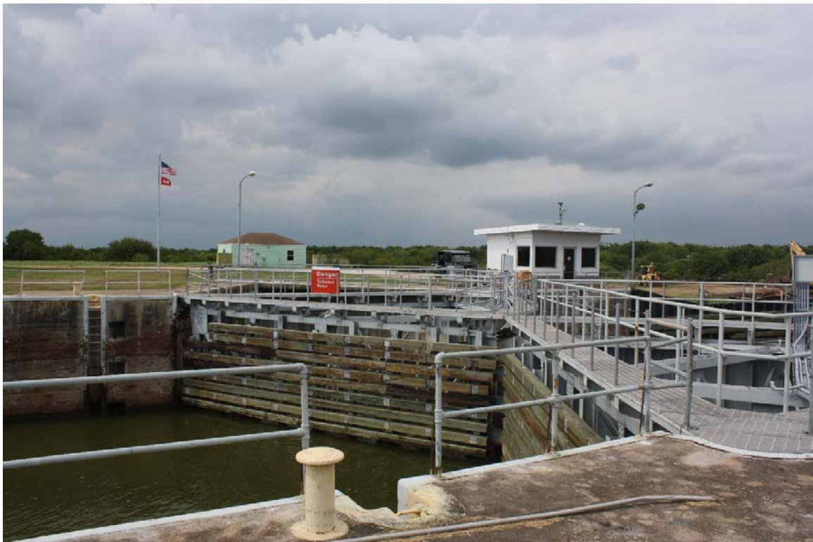
View showing relationship between 1944 control house and power house, facing north
