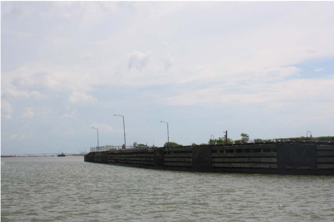
View of south guide wall, facing east
