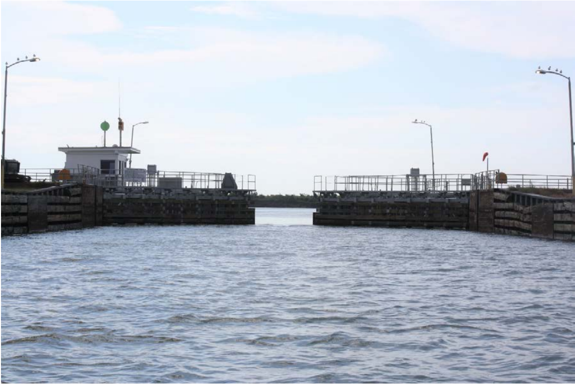
Representative view of floodgates in process of opening, facing northeast
