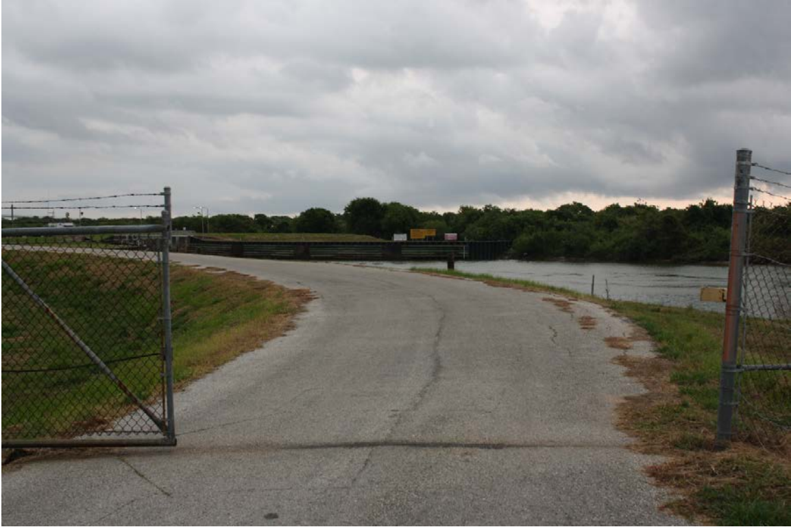
D25: View of entrance to east locks, facing southeast
