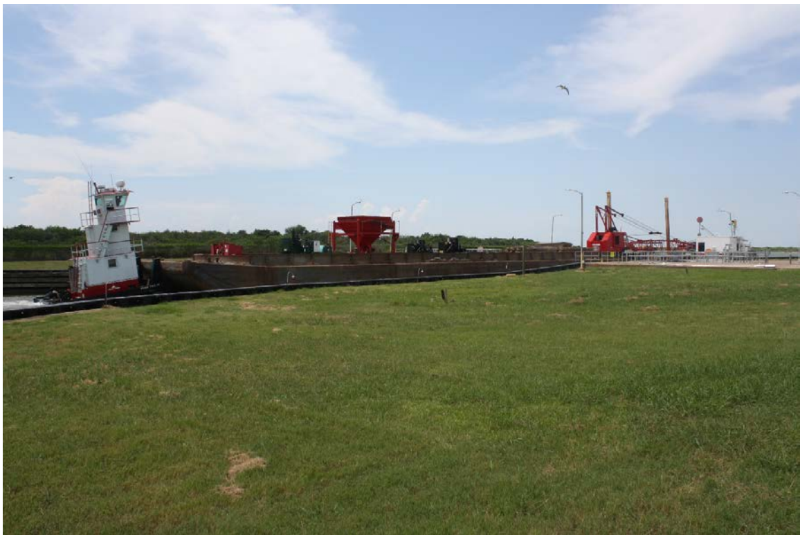
D16: View of barge traveling west through the east floodgate, facing south
