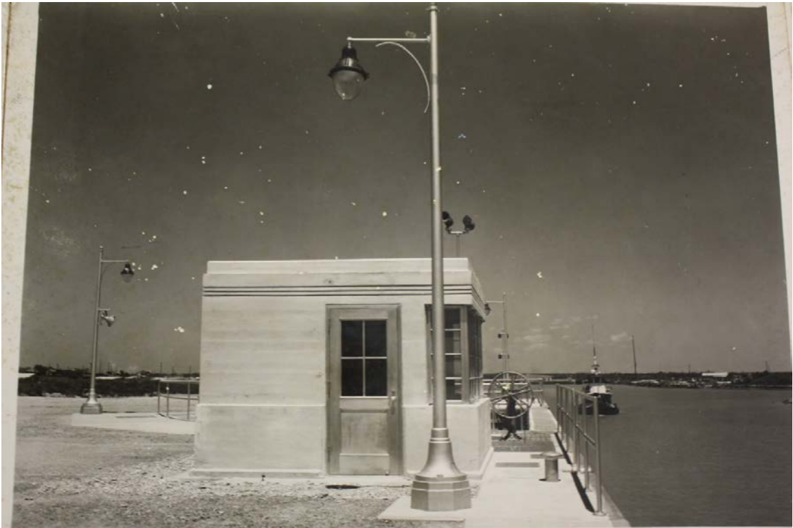
Photo dated 1954 showing the 1951 control house, facing northeast
