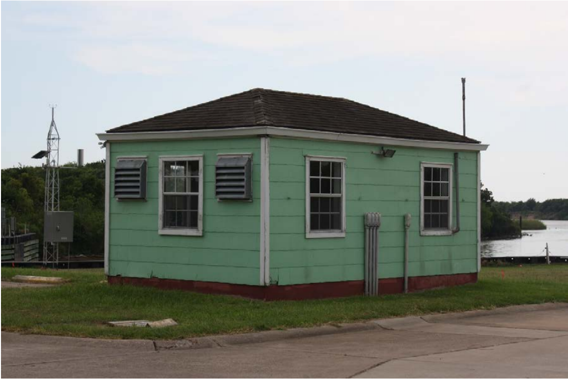
Oblique view, facing southwest
