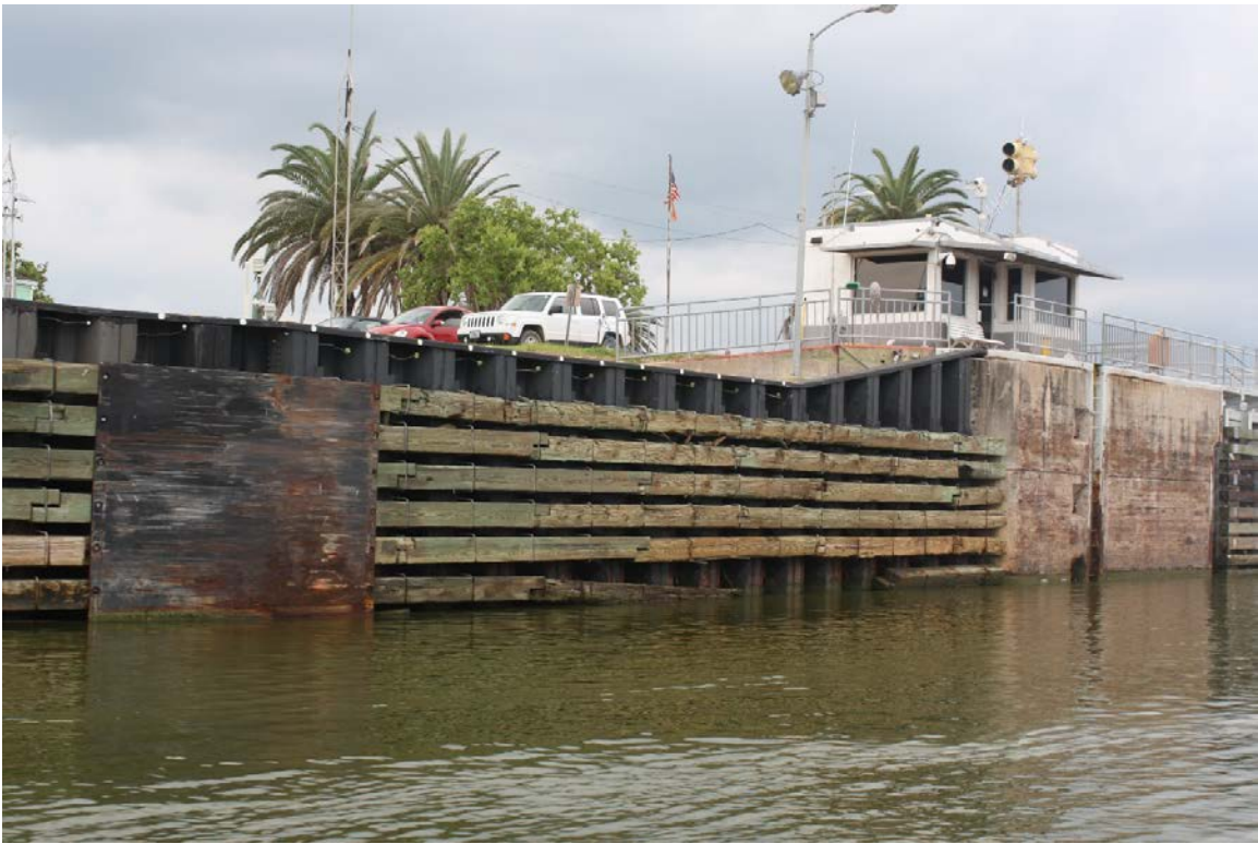
Representative view of damage to timber guide walls, facing west
