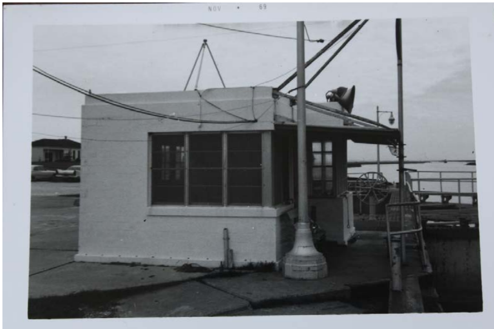
Photo from 1969 showing original multi-light windows, facing northeast. Image courtesy of USACE.
