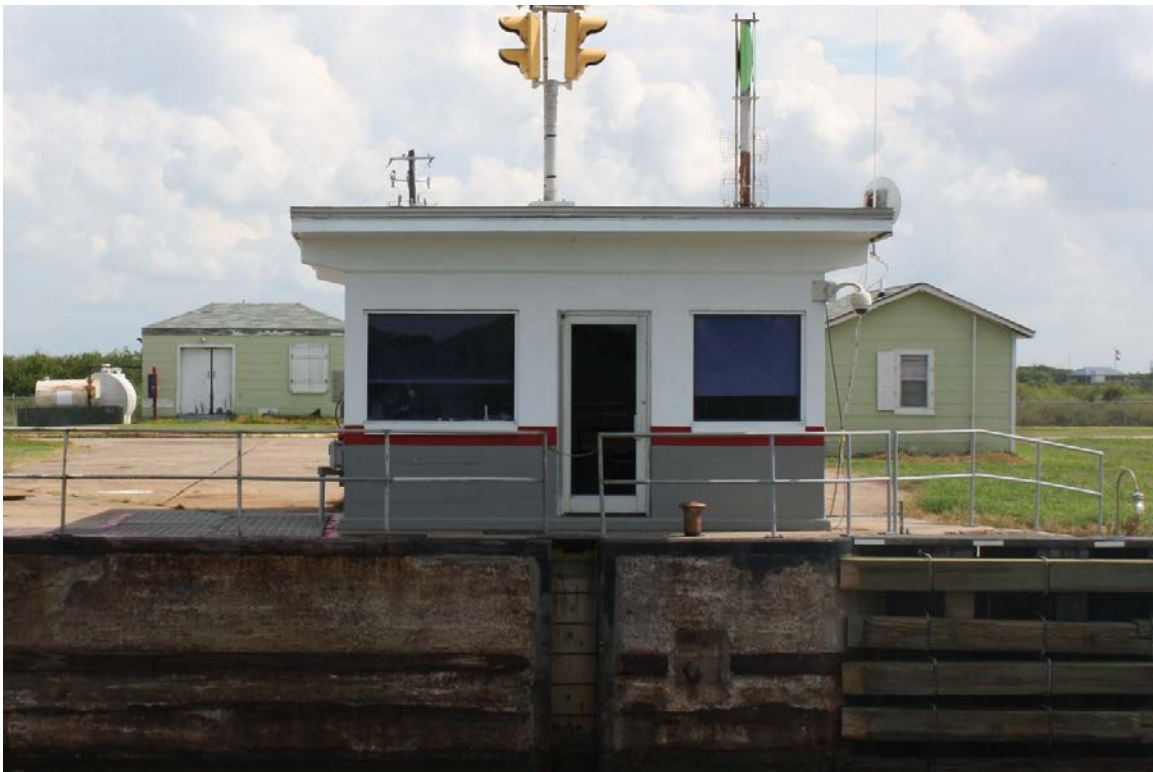
View of Brazos River west floodgate control house, facing north
