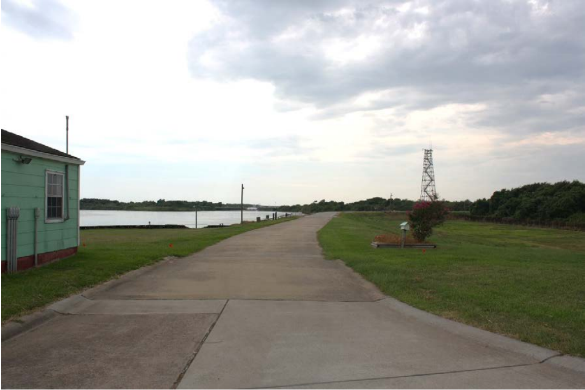
D27: View of internal access road toward entrance gate, facing west. The power house (Resource No. 15) is on the left.
