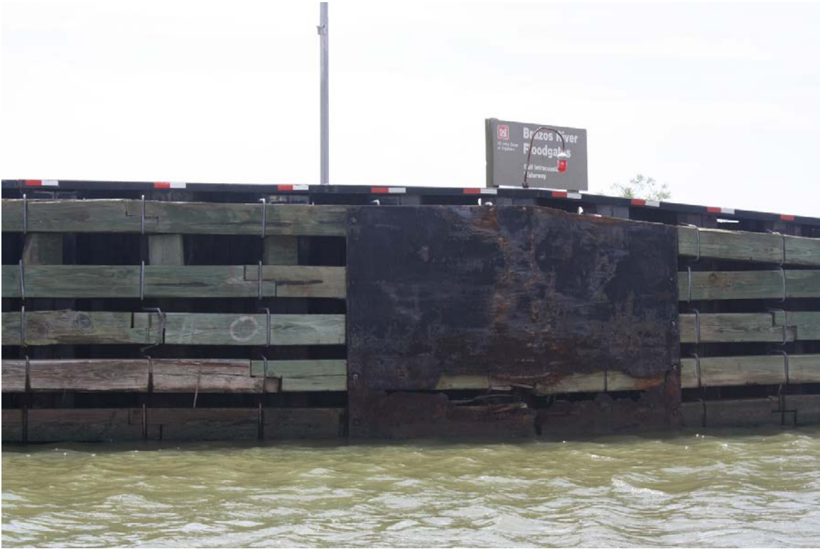
Representative view of section loss and impact damage to steel sheets, facing east
