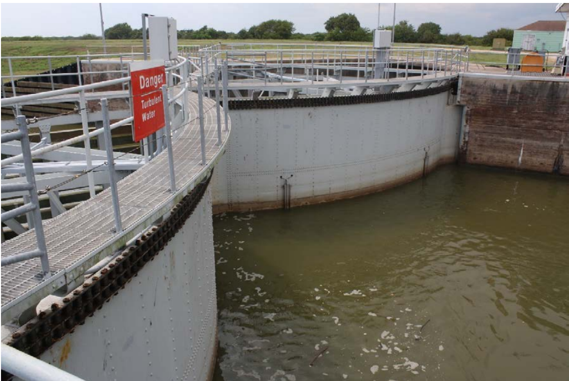
Representative photo of closed lock gates, facing northwest
