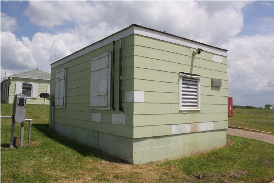
Oblique view, facing north. Resource No. 7 is in the background.
