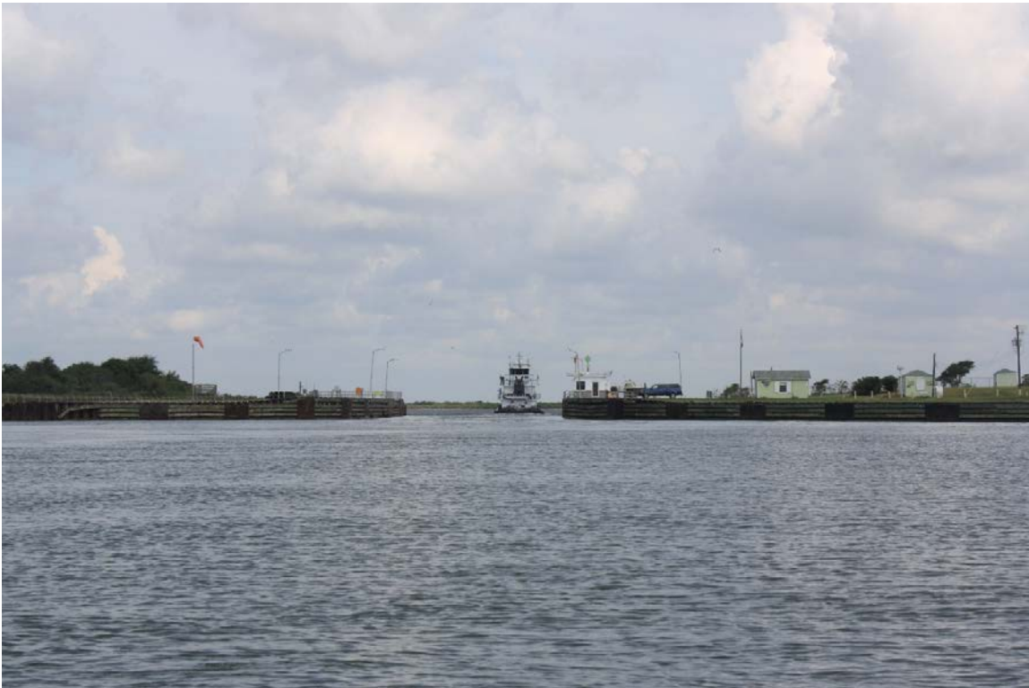
Overall view of west Brazos River floodgate, facing northwest
