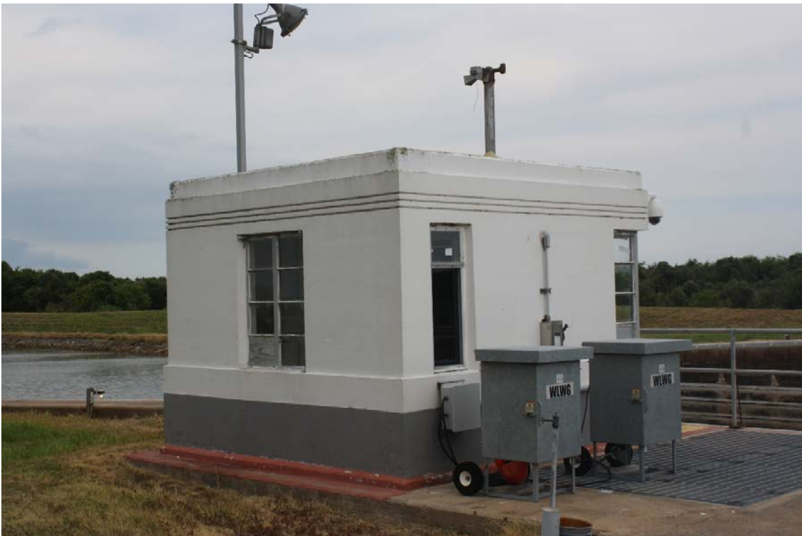
View of rear (north) and west elevation, facing east
