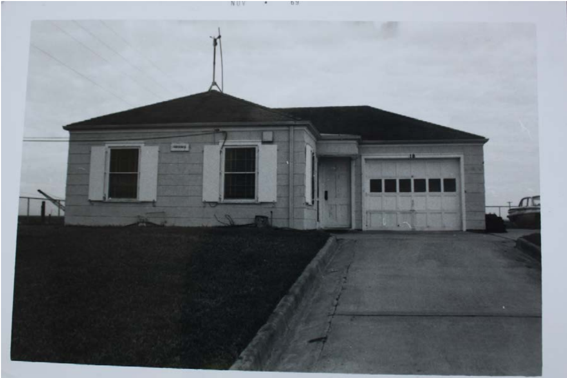
Photo dated 1969 showing front (south) elevation of office, facing northwest. Garage access door has since been infilled. Image courtesy of USACE.
