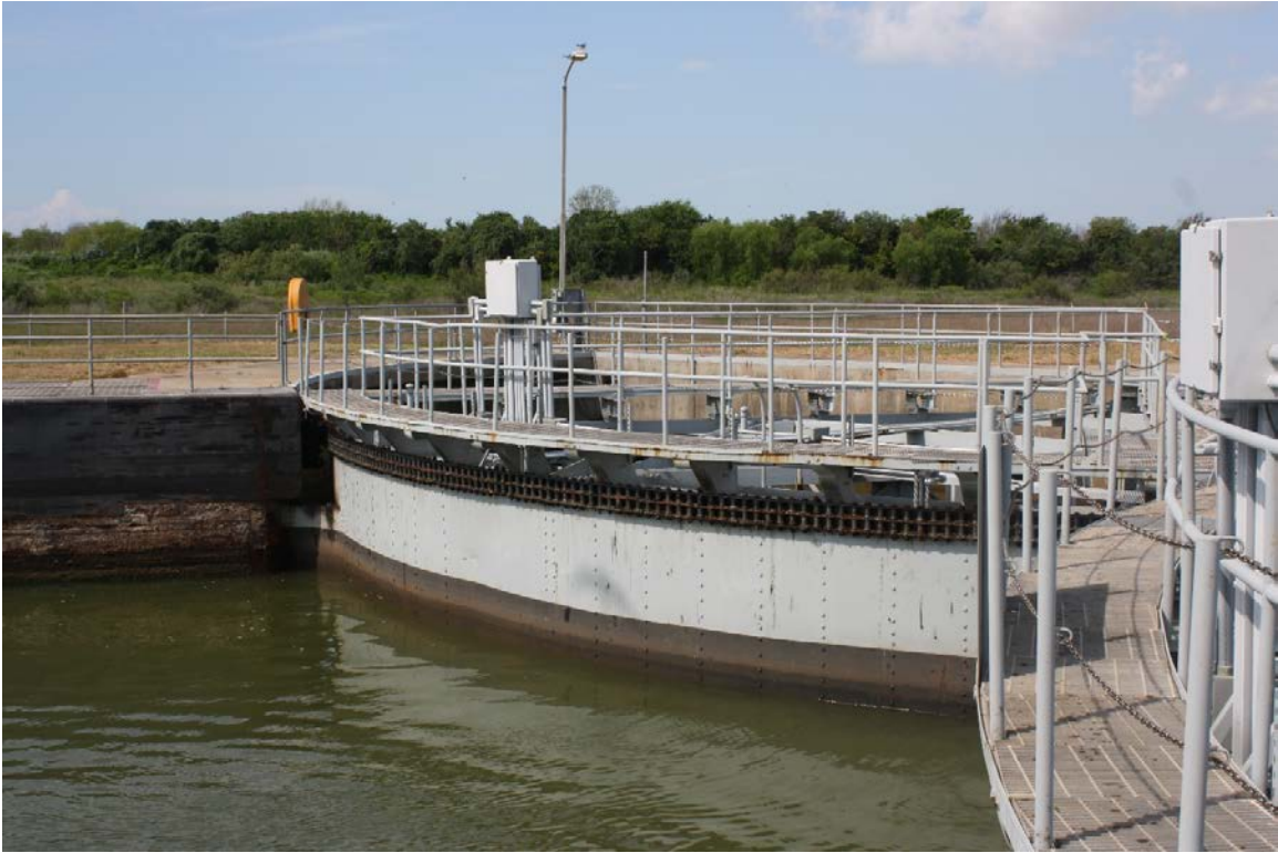
Representative view of closed gate, facing south.
