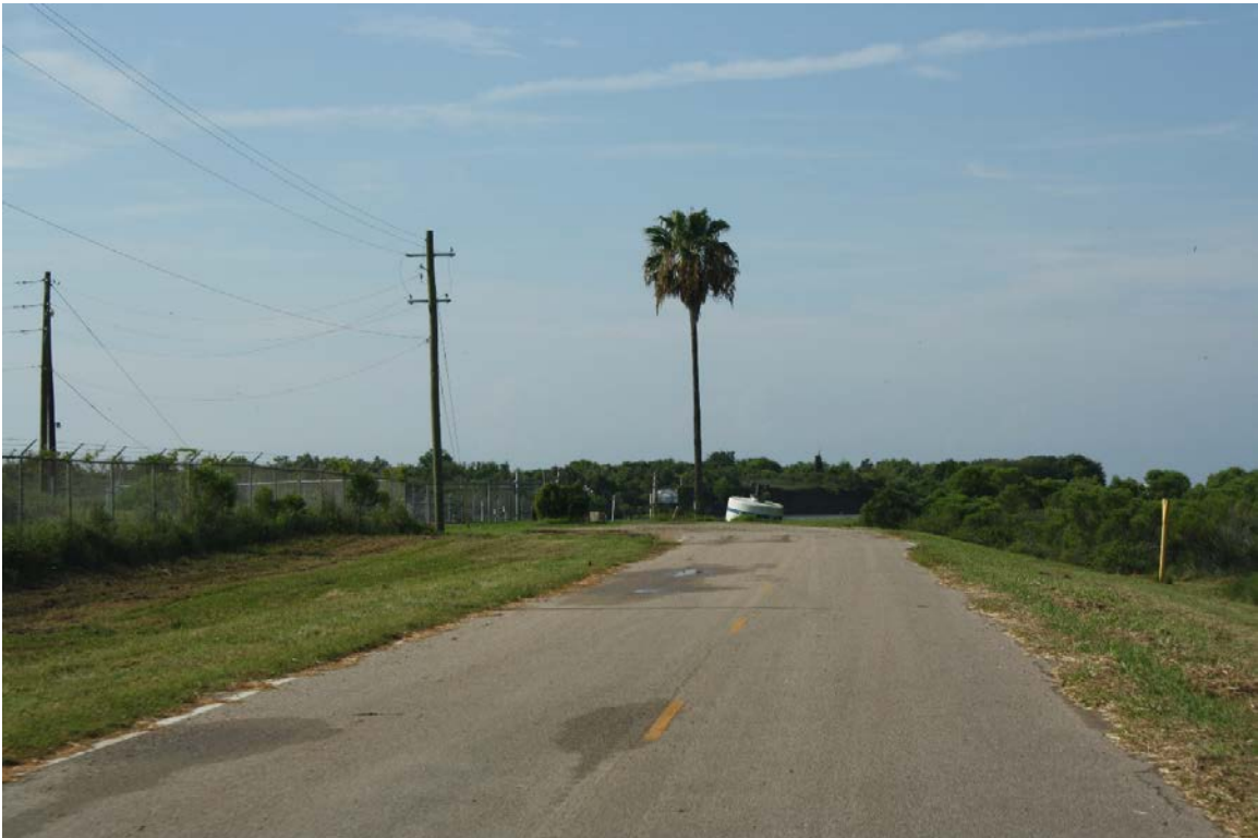
D10: View toward east floodgate entrance gate, facing southeast
