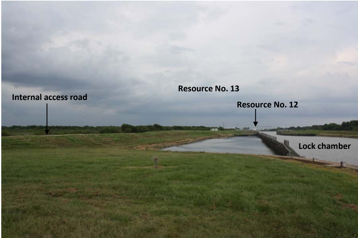
D19: View from 1951 control house toward 1944 control house (Resource Nos. 11 and 12), facing northwest
