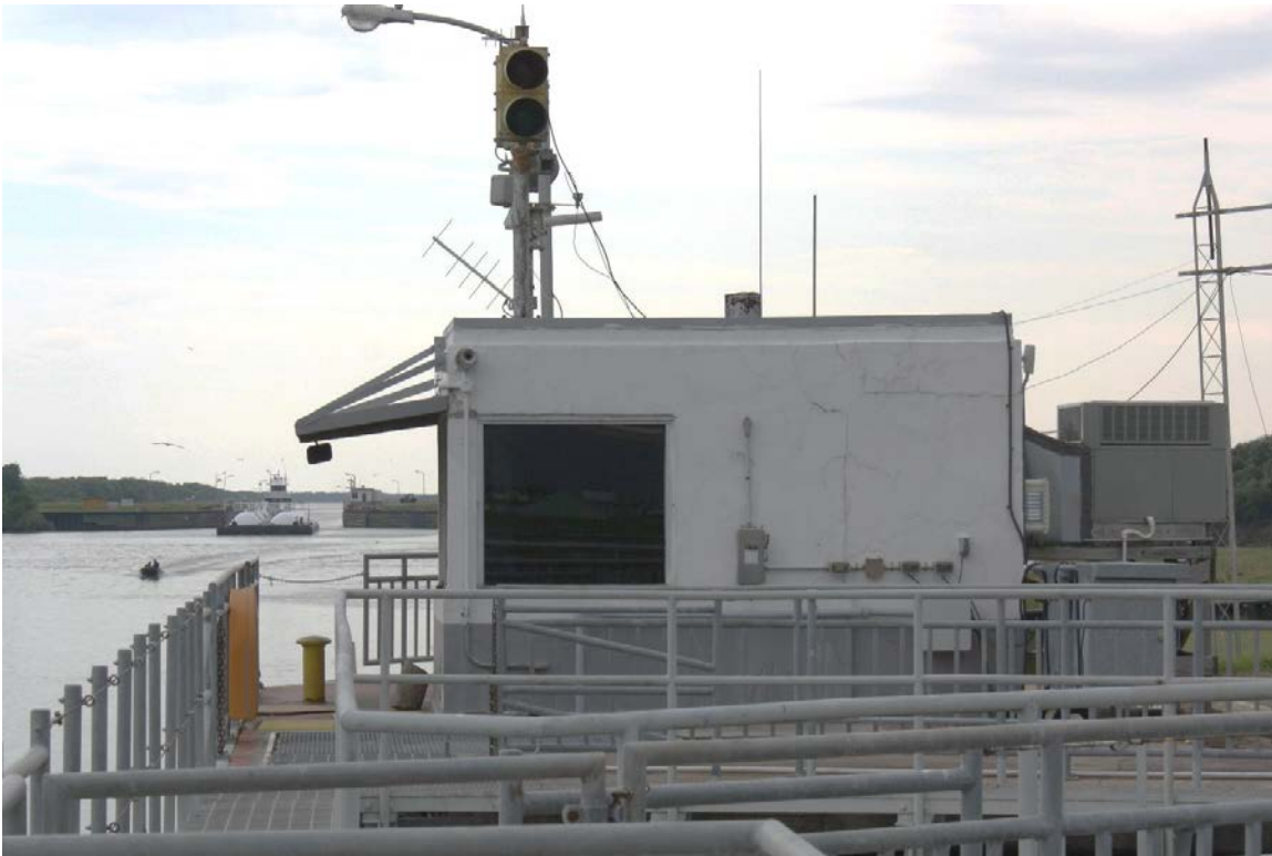
View of east elevation, facing southwest
