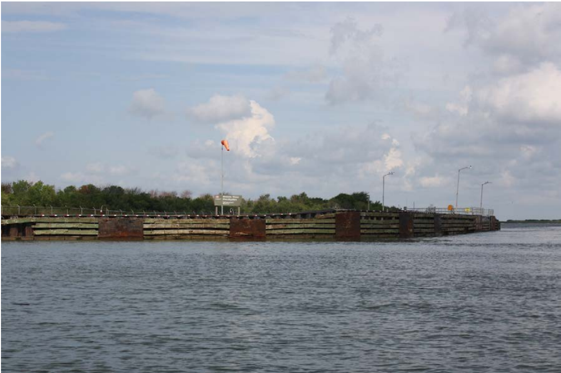
View of south guide wall, facing west
