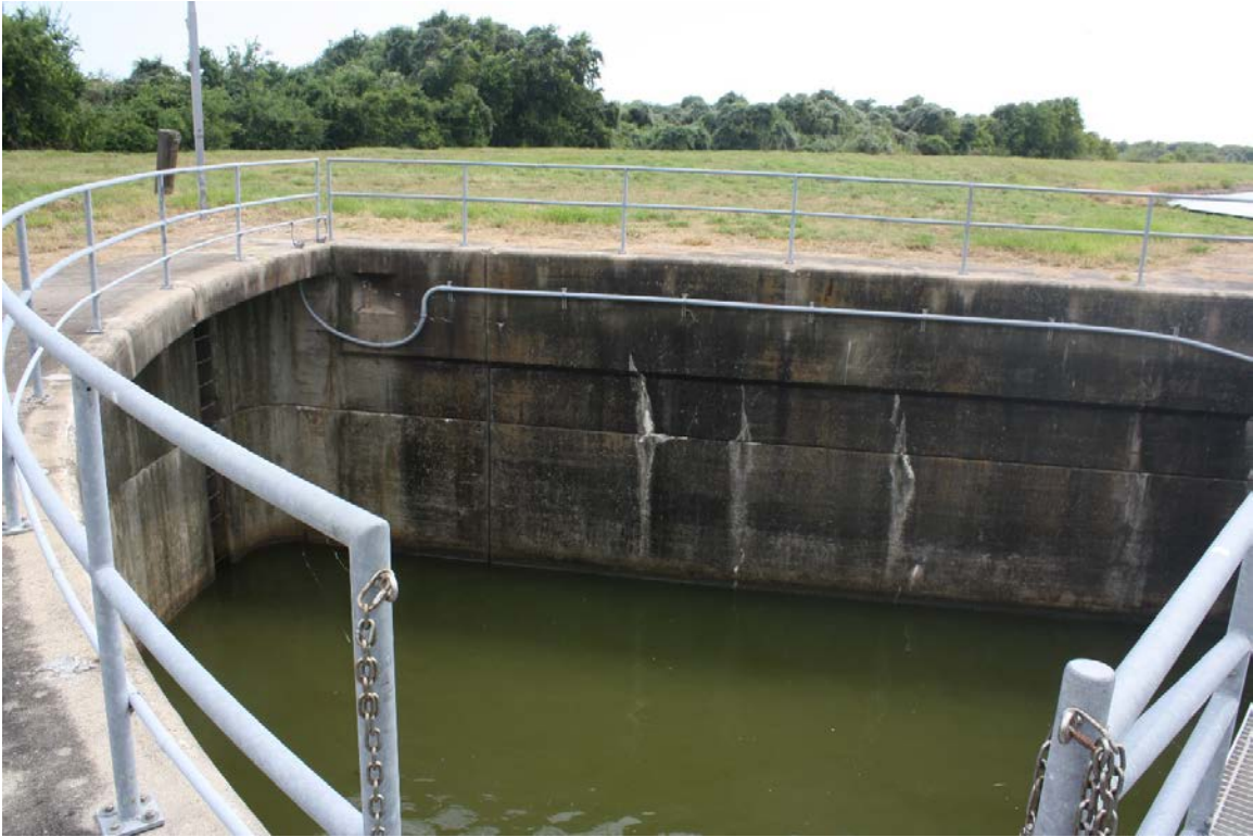
Representative photo of lock concrete recess well, facing southwest
