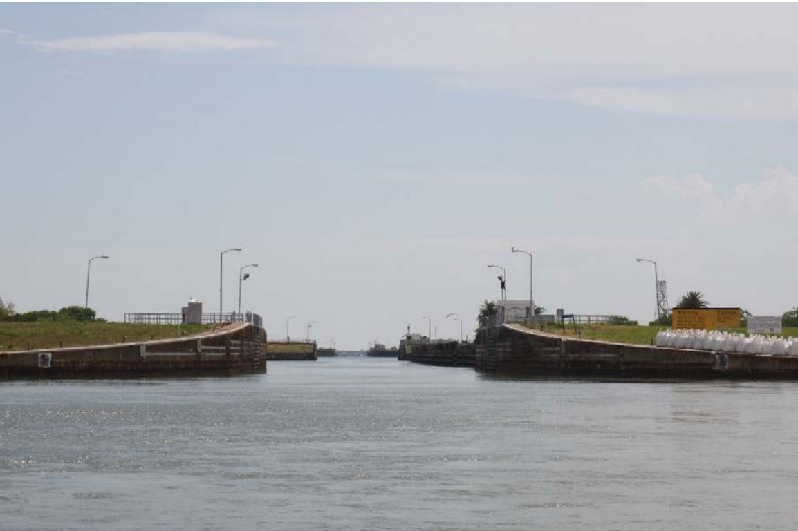
View of east lock guide walls, lock gates, and lock chamber, facing southwest
