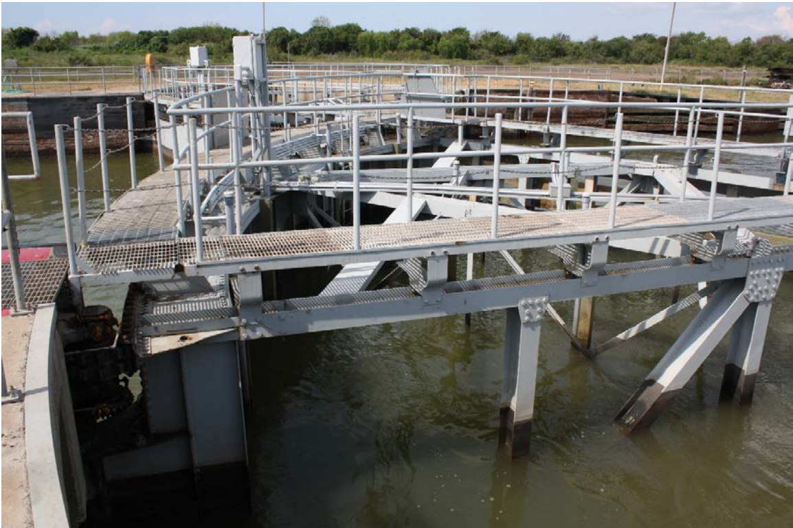
Representative view of gate from recess well, facing south
