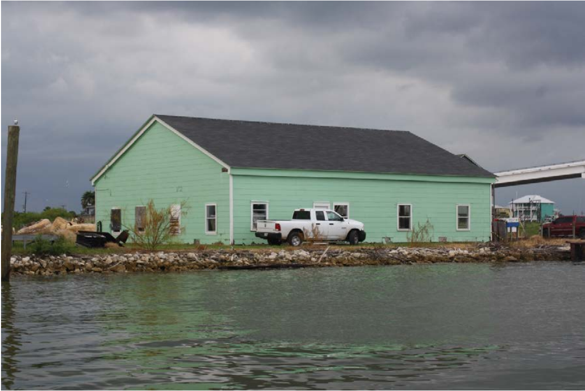
View of boat house from GIWW, facing northwest
