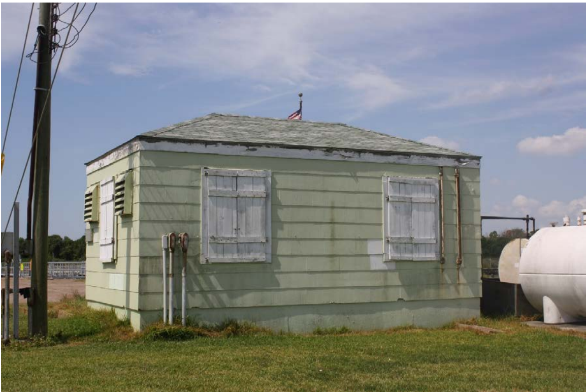
View of north elevation, facing southwest
