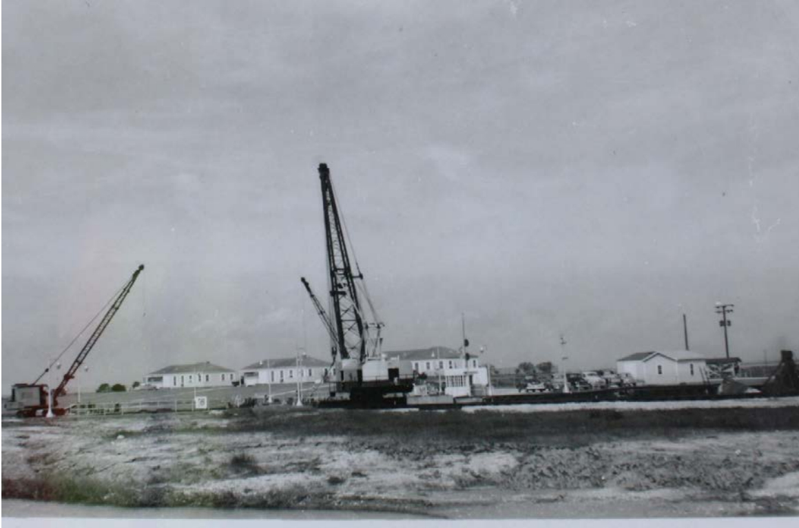
D5: Photo from the early 1940s showing the no longer extant three residences on the west floodgate, facing north. Photo courtesy of USACE.
