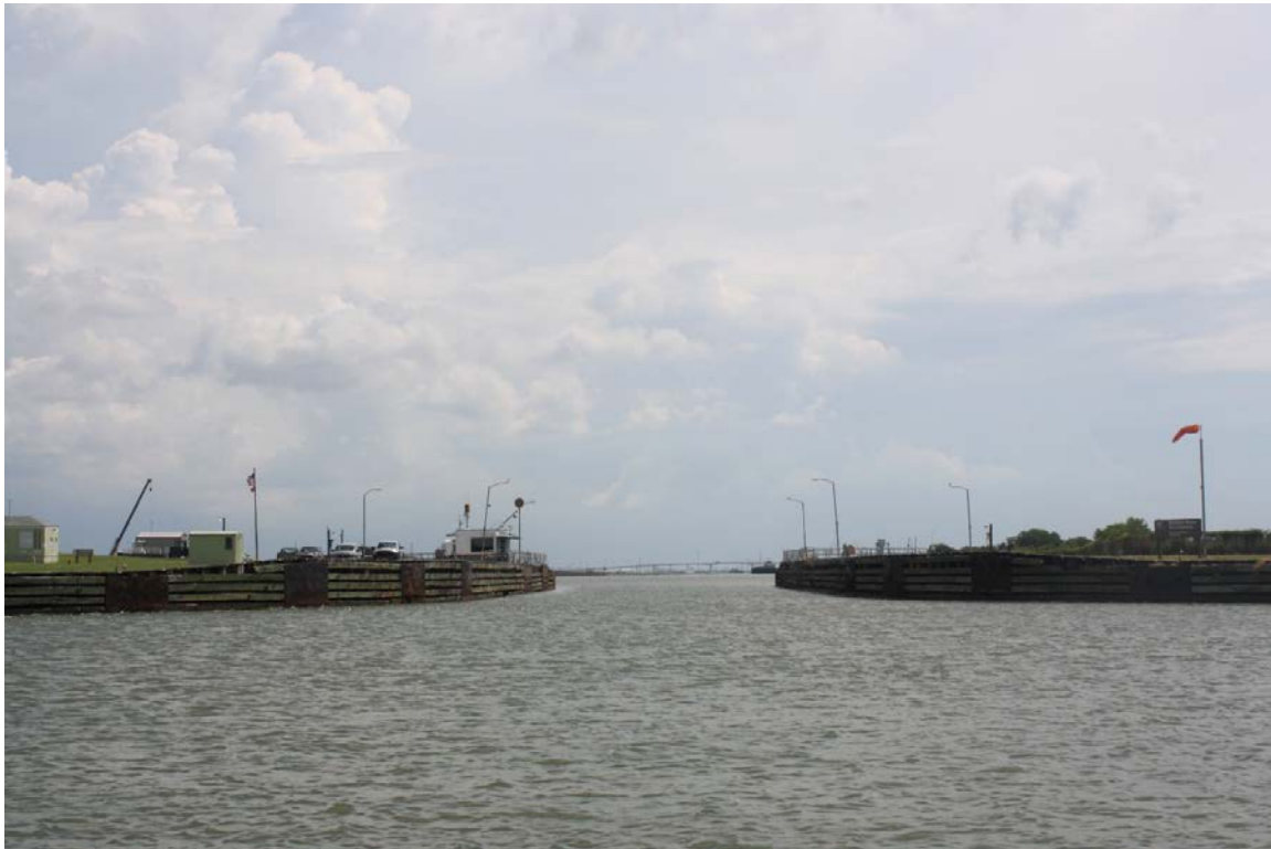
Overall view of east Brazos River floodgate, facing northwest
