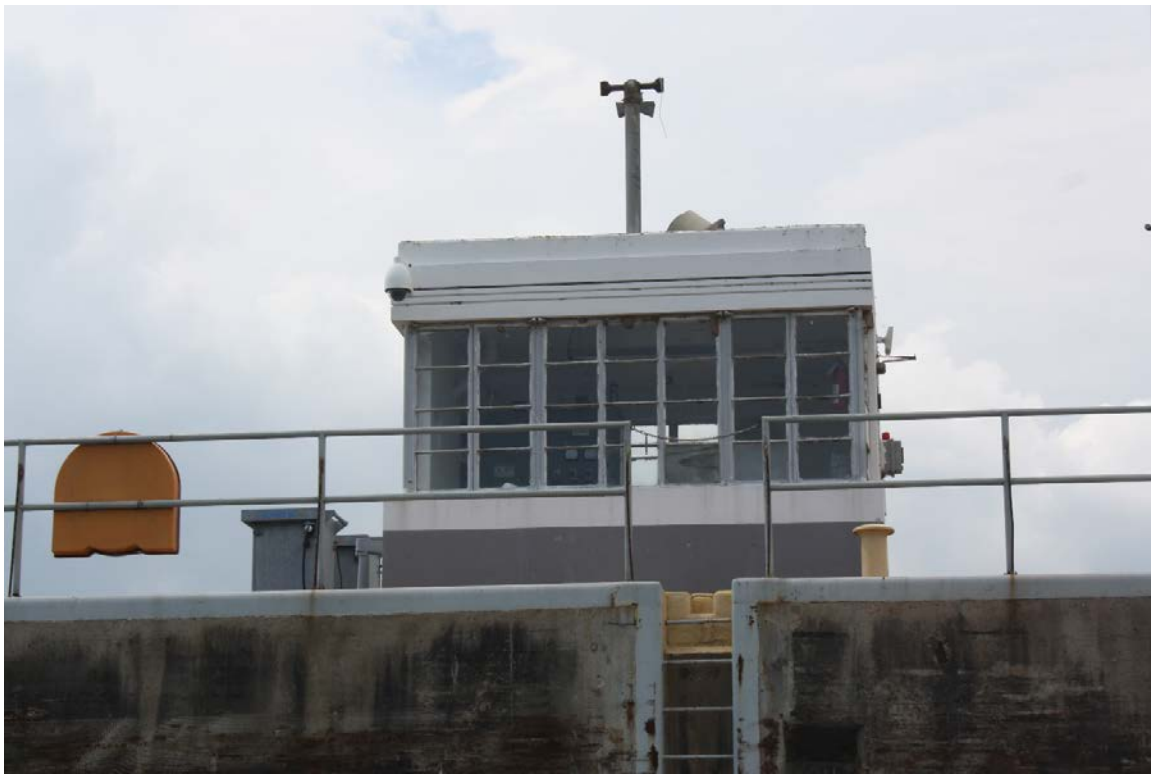
View of control house from GIWW, facing north
