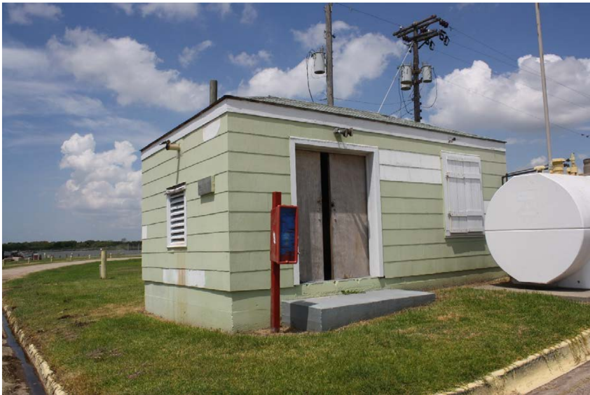
Oblique view, facing west
