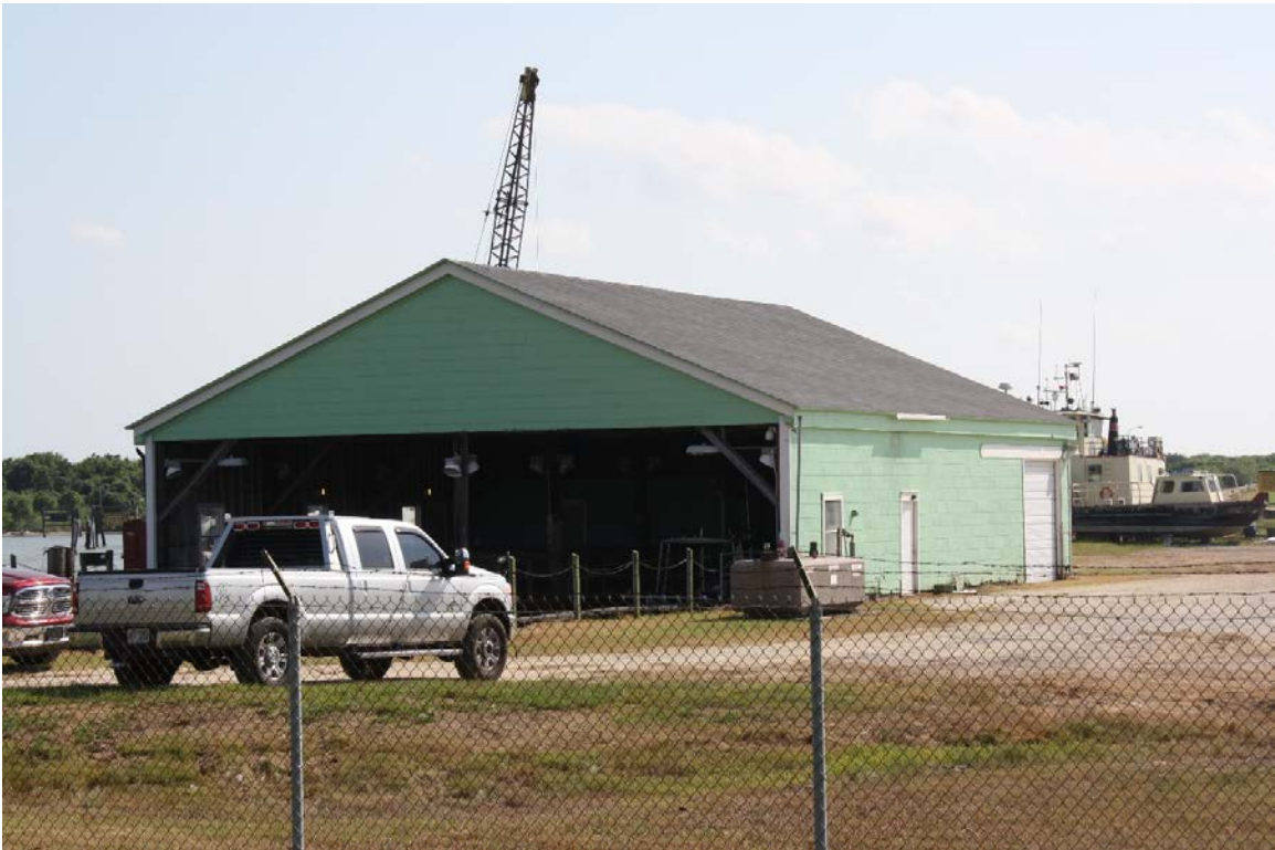
View of boat house, facing west
