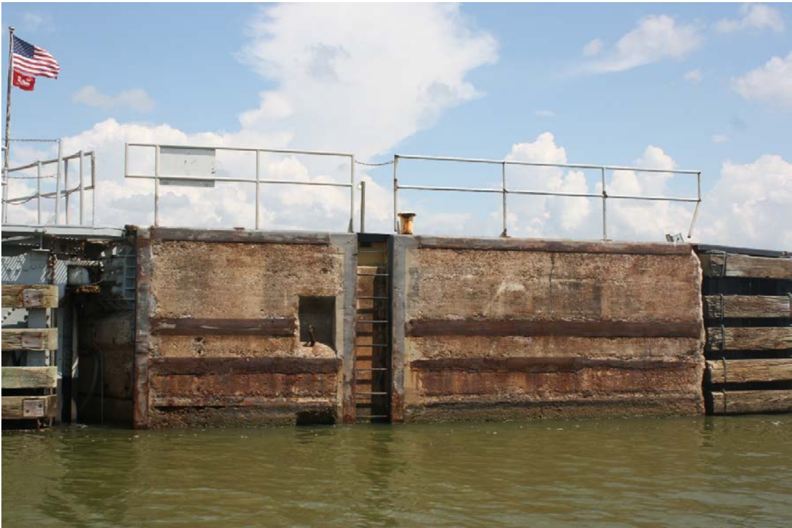
Representative view of cracked and spalling concrete, facing north
