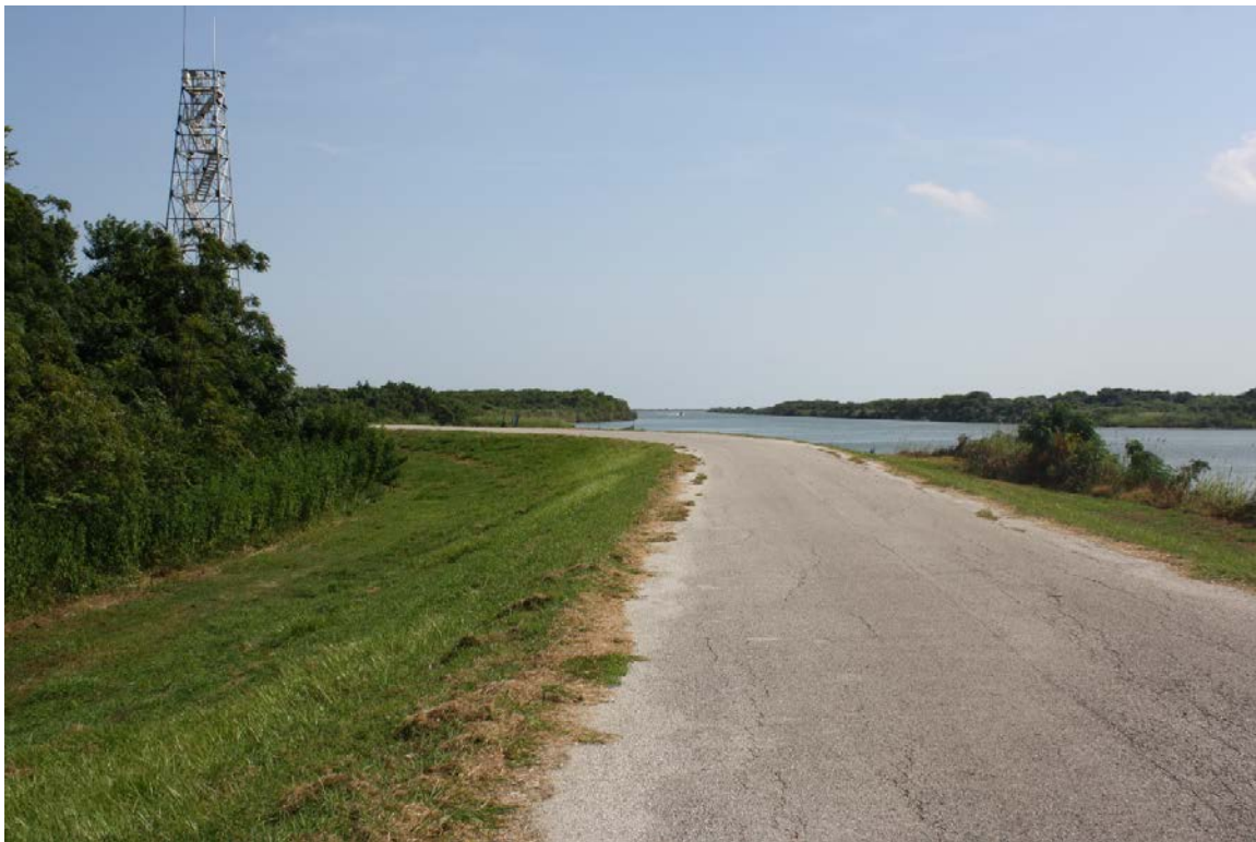
D24: View of west lock access road toward entrance, facing south.
