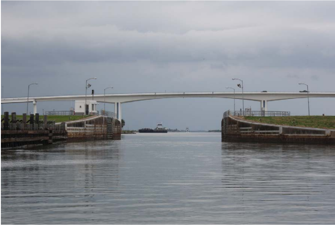
View of 1951 guide walls and lock gates from lock chamber, facing northeast
