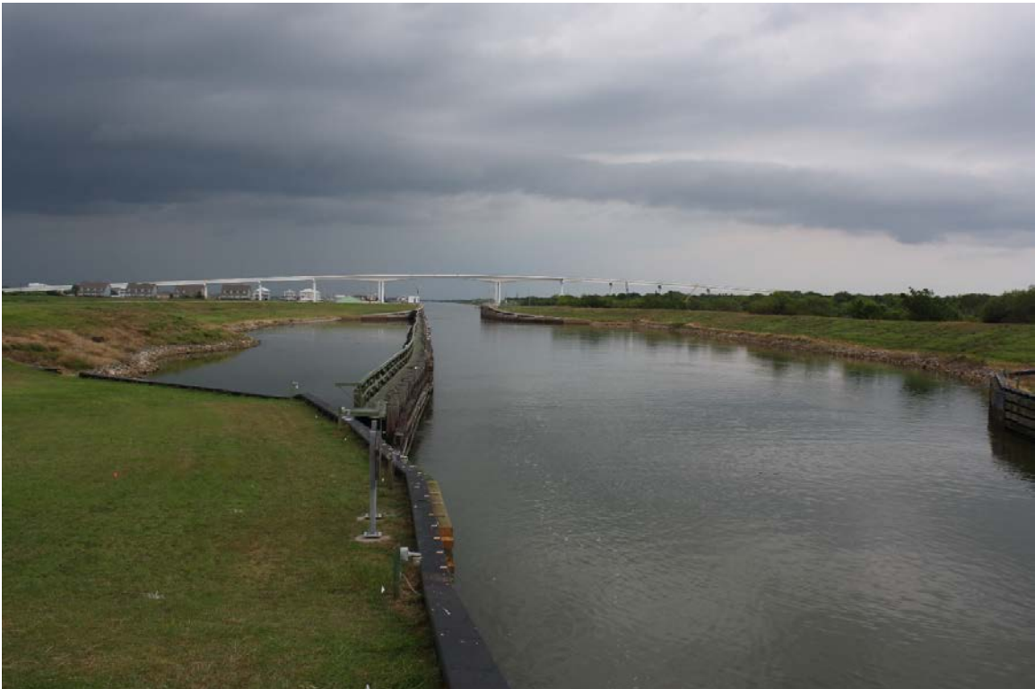
View of lock chamber, facing northeast
