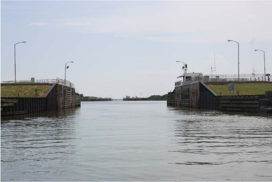
View of 1944 lock gates, facing southwest toward Colorado River
