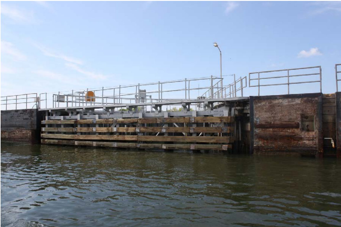
View of south gate, facing south
