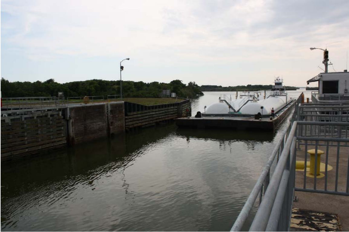
D35: View of barge traveling east through east locks, facing southwest
