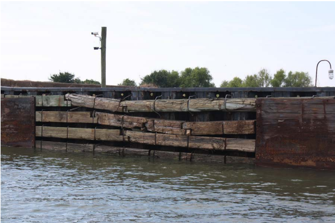
Representative view of damage to timber fenders, facing north
