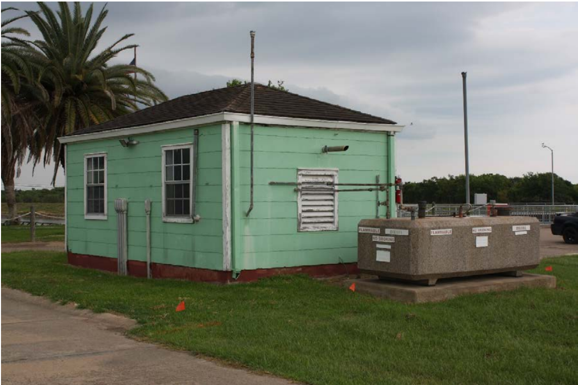
Oblique view, facing east
