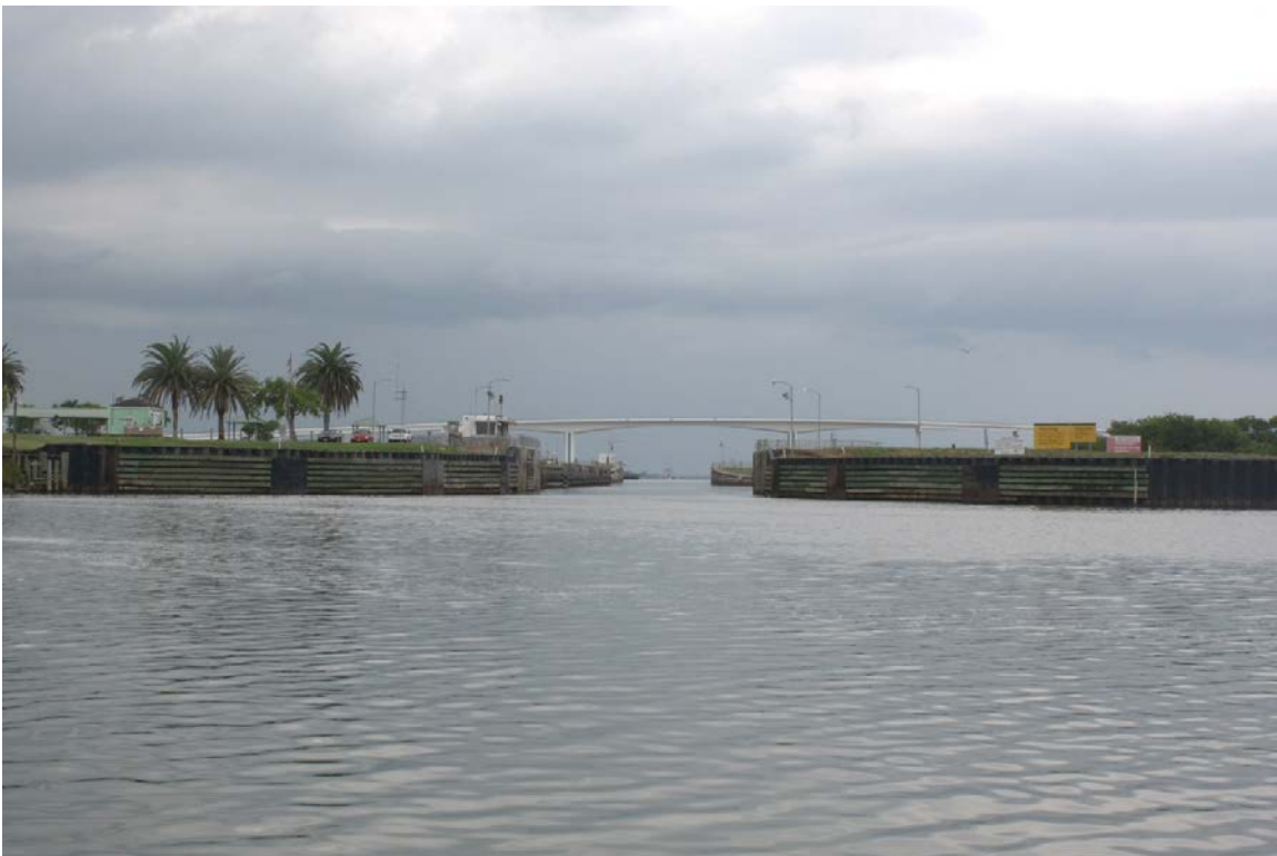
View of east lock guide walls, lock gates, and lock chamber, facing northeast from the Colorado River
