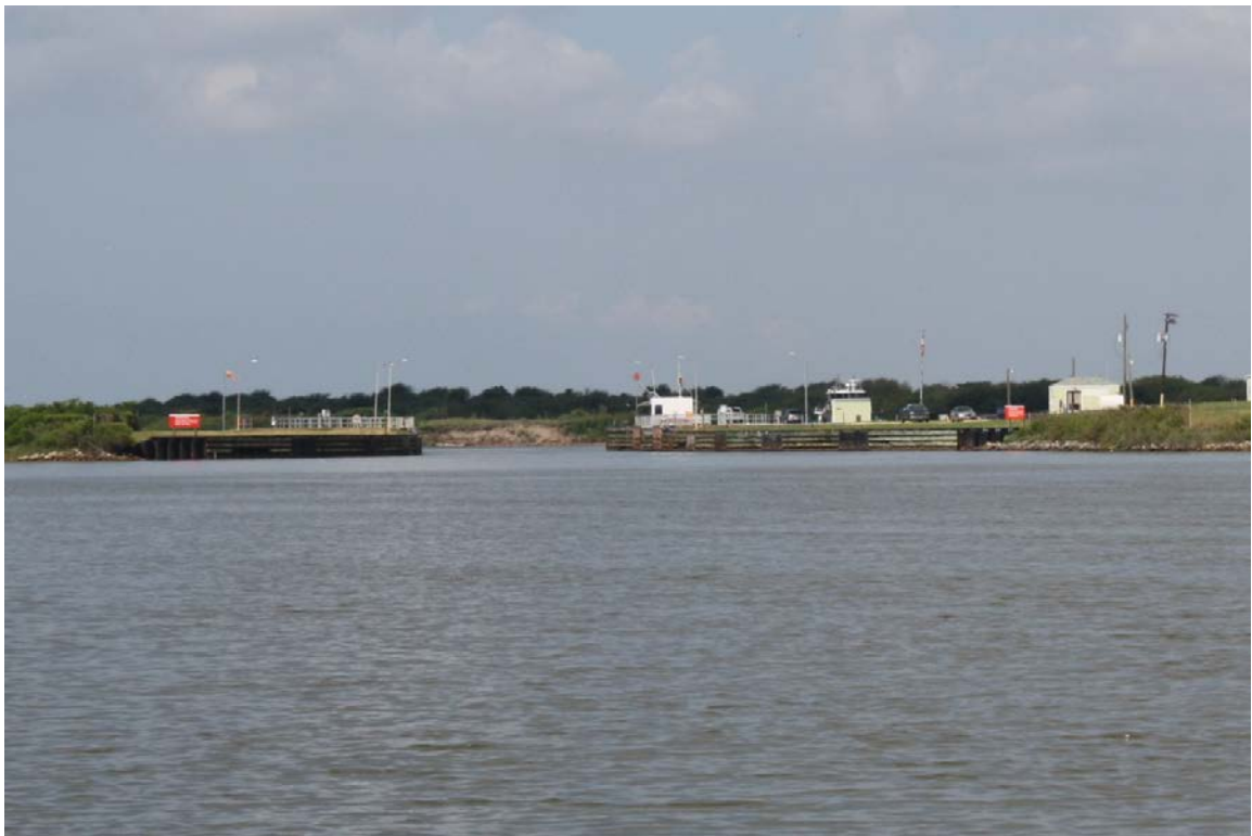
View of east floodgates and buildings from GIWW, facing southwest
