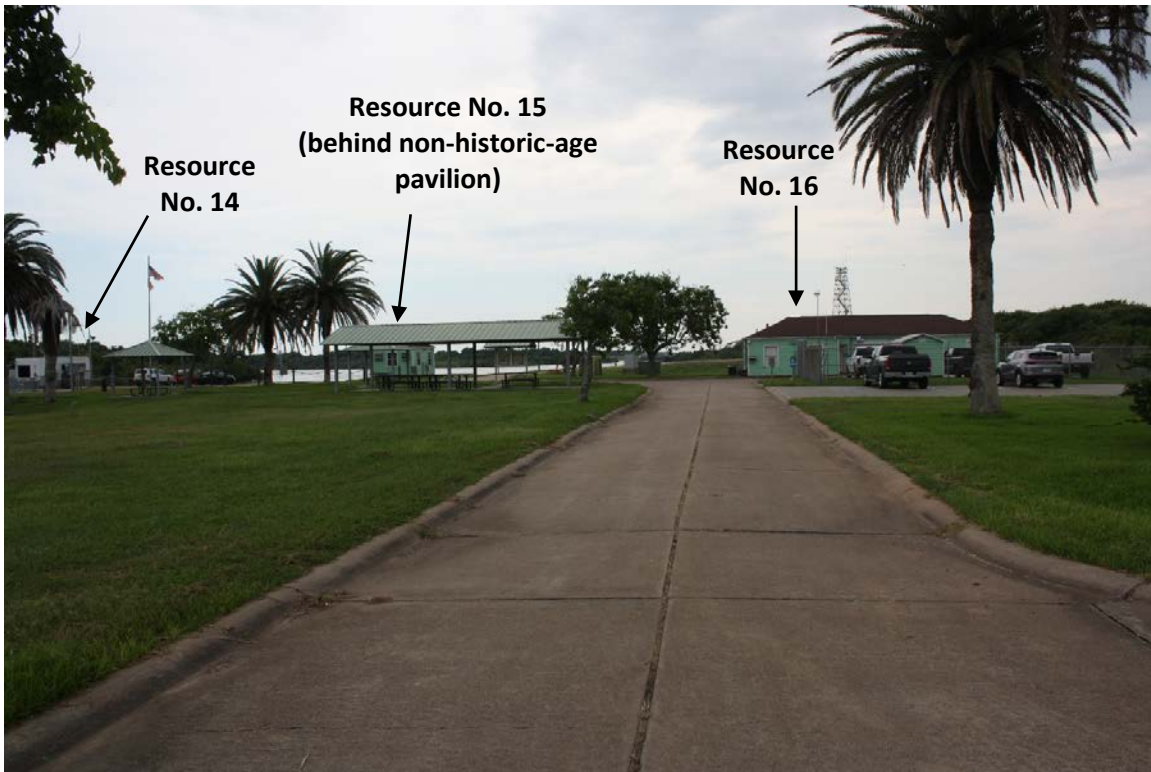
D29: View of internal access road toward office and power and control houses (Resource Nos. 14-16, respectively), facing southeast. Grassy area on both sides of road originally had six total residences.
