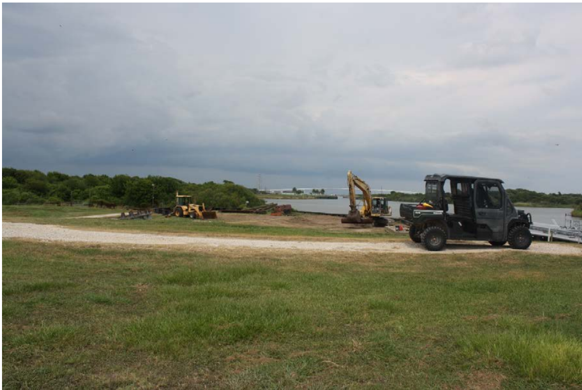
D18: View from 1944 control house (Resource No. 12) toward Colorado River and east locks, facing east
