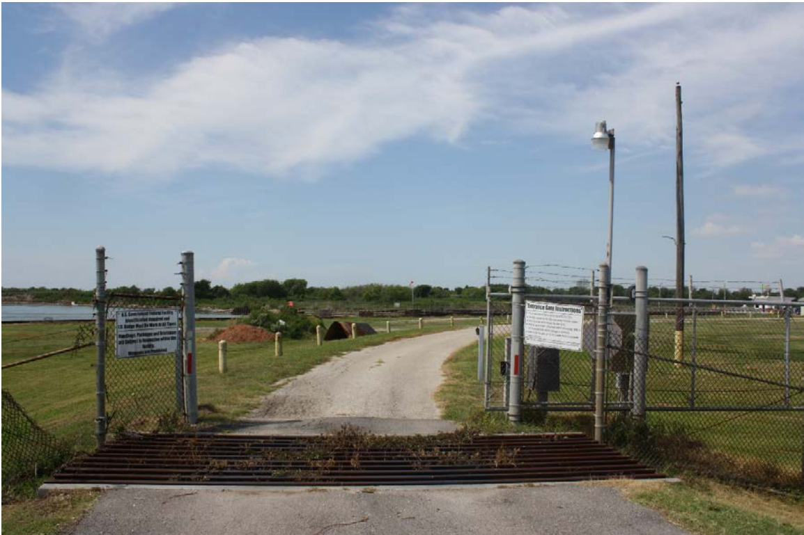
D2: View of west floodgates entrance gate, facing southeast toward the GIWW
