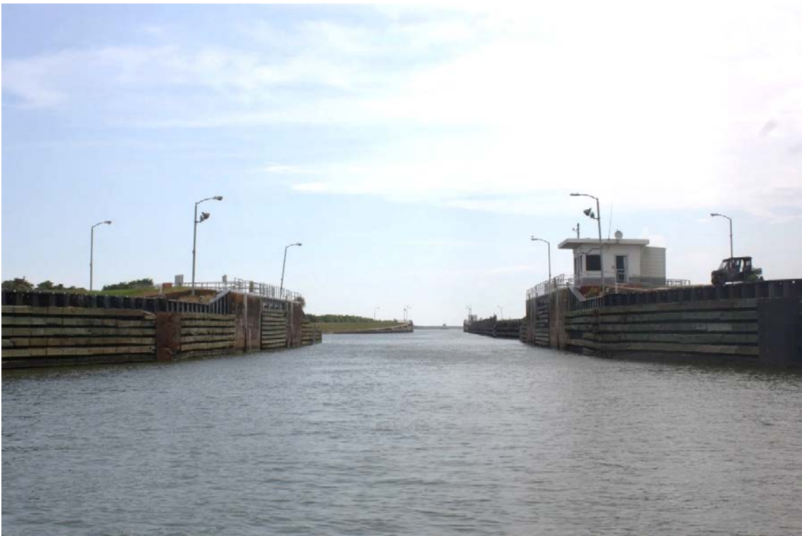
View of 1944 guide walls, lock gates, and lock chamber, facing southwest
