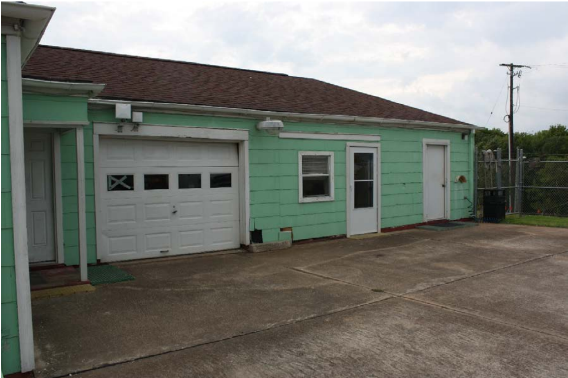
View showing converted garage space, facing west
