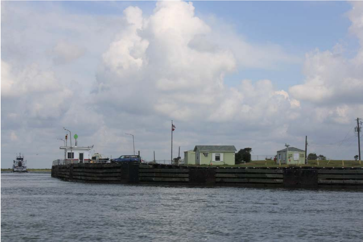
View of north guide wall, facing northwest. Resource Nos. 2-4 include control house and sheds.
