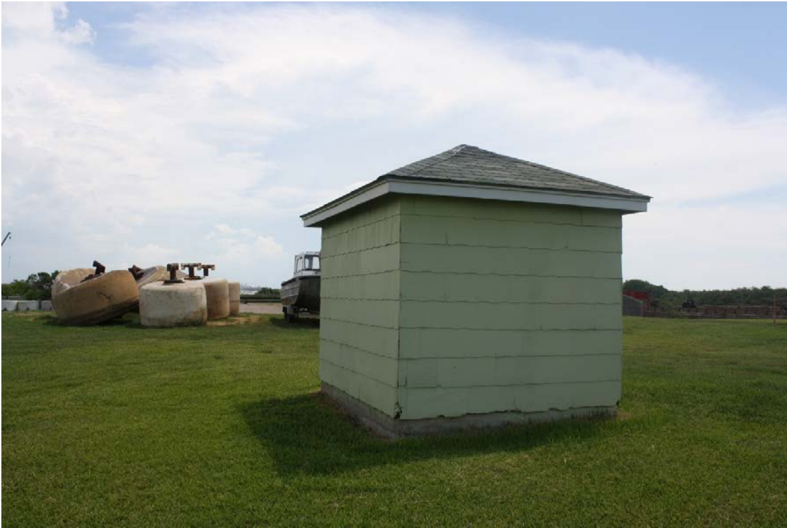
View of rear (north elevation), facing south
