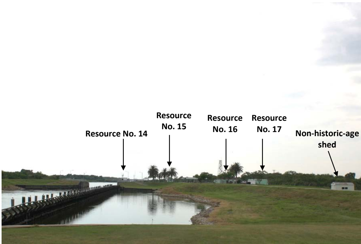
D31: View from 1951 control house (Resource No. 18) toward 1944 control house (Resource No. 14), facing southwest.
