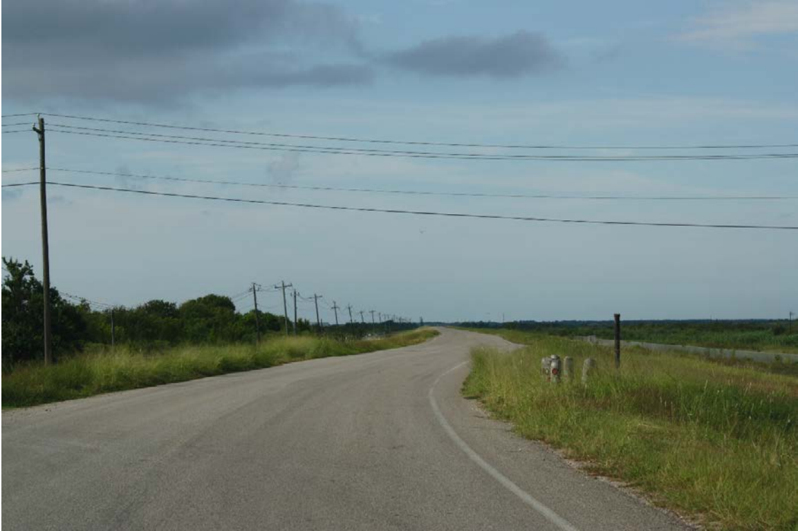
D9: View of east floodgate access road from SH 36, facing southwest. Access road is 3.4 miles in length
