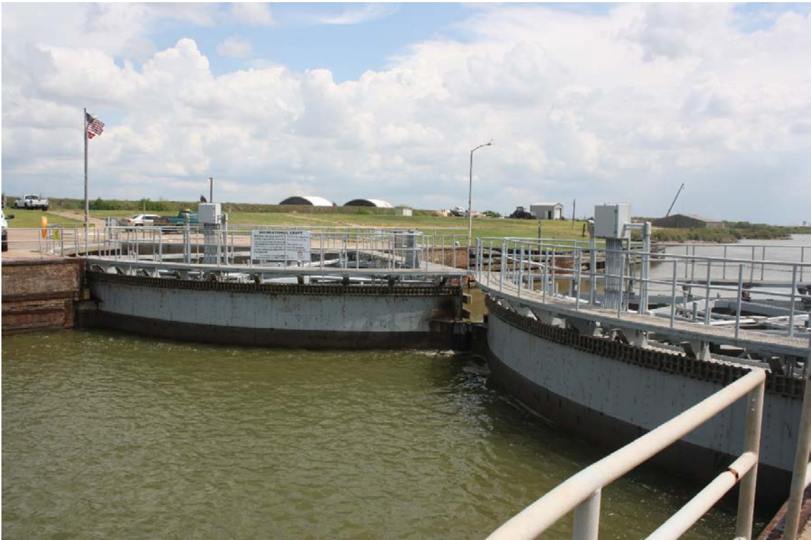
Representative view of closed gates, facing northeast
