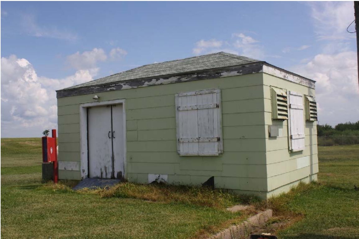
Oblique view, facing north
