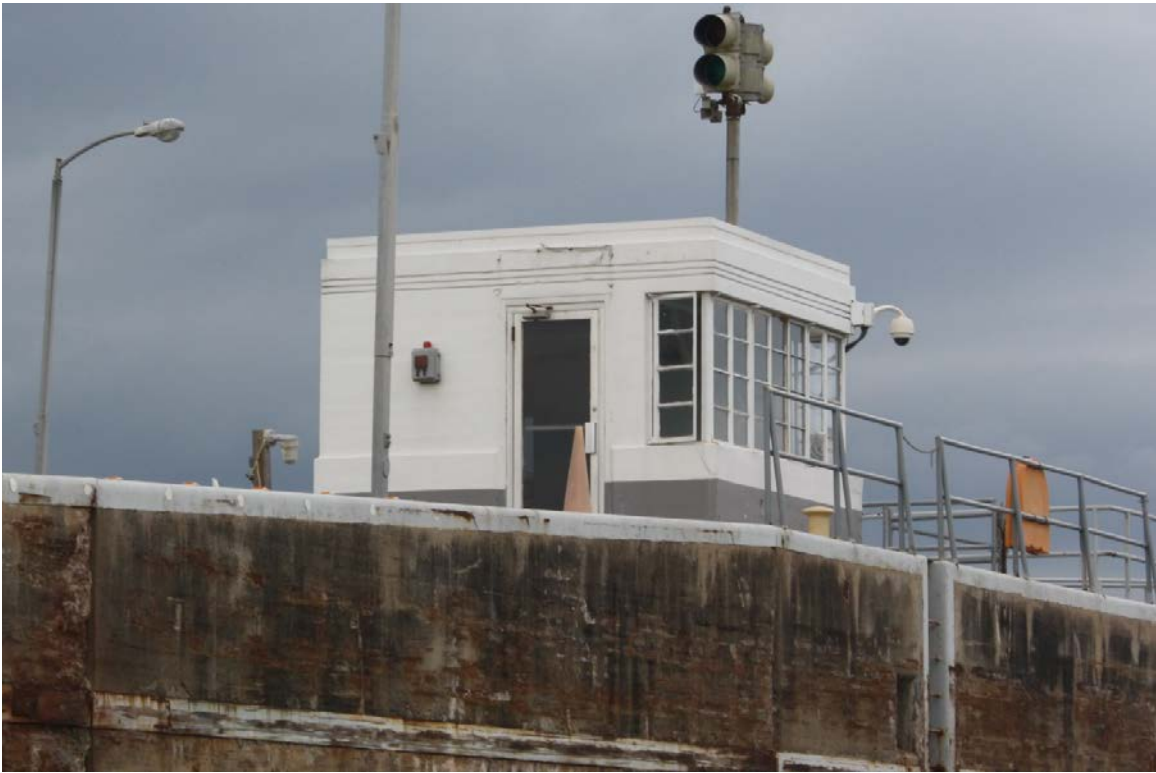
View of 1951 control house, facing northeast
