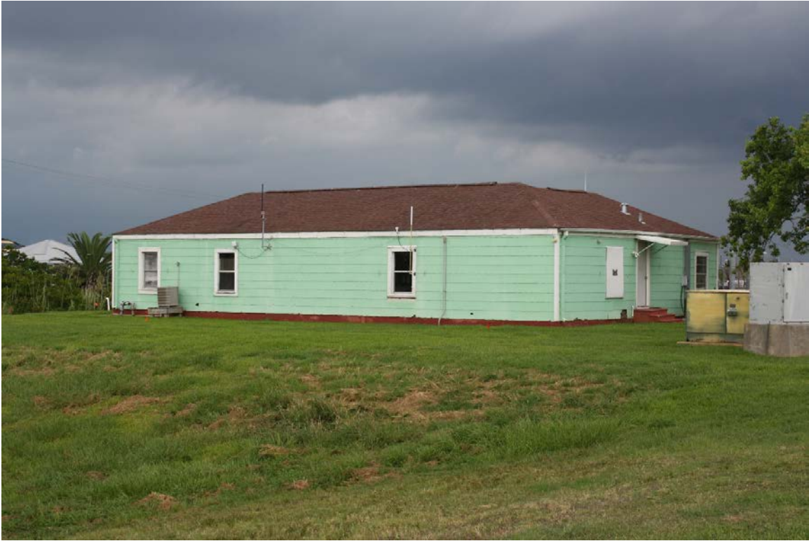
Oblique view, facing northeast
