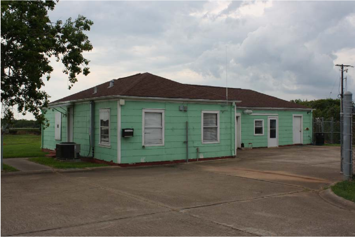
Oblique view, facing west
