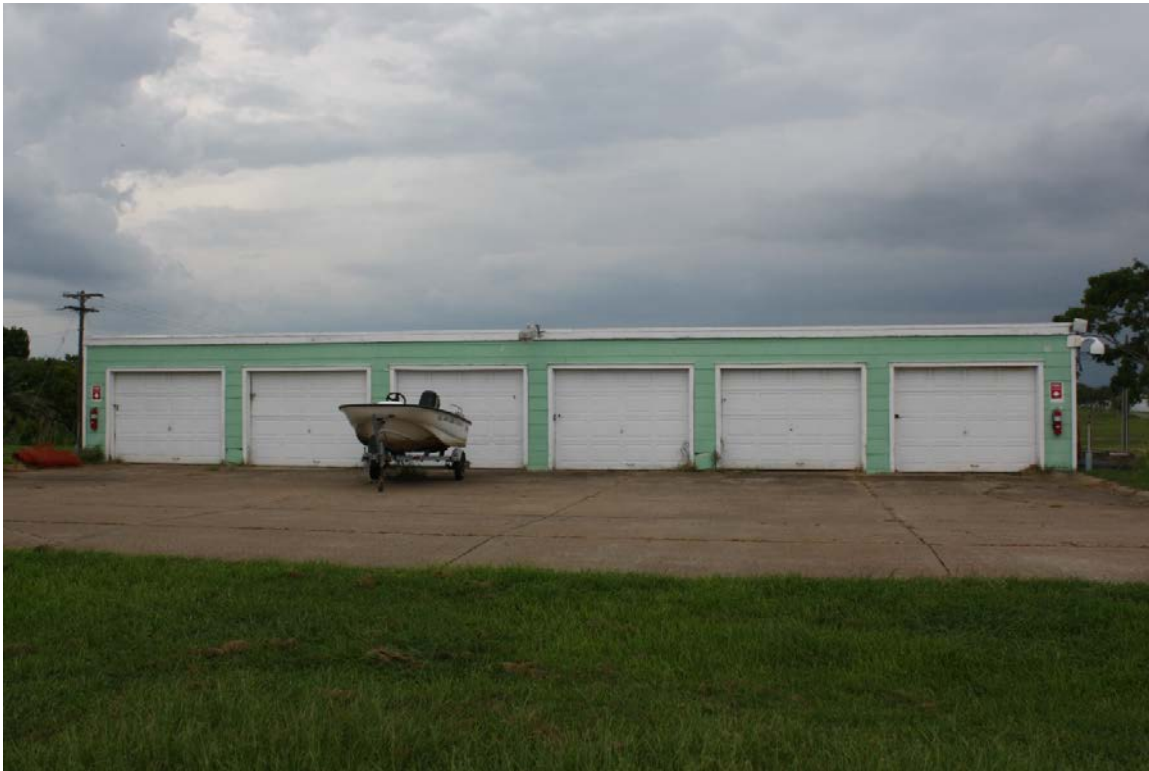
View of south elevation of garage, facing northwest
