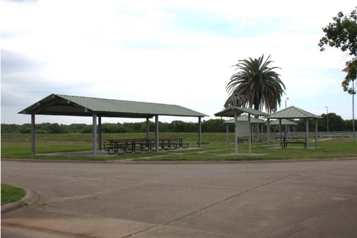
D28: View of non-historic-age pavilions just north of 1944 control house, facing southeast
