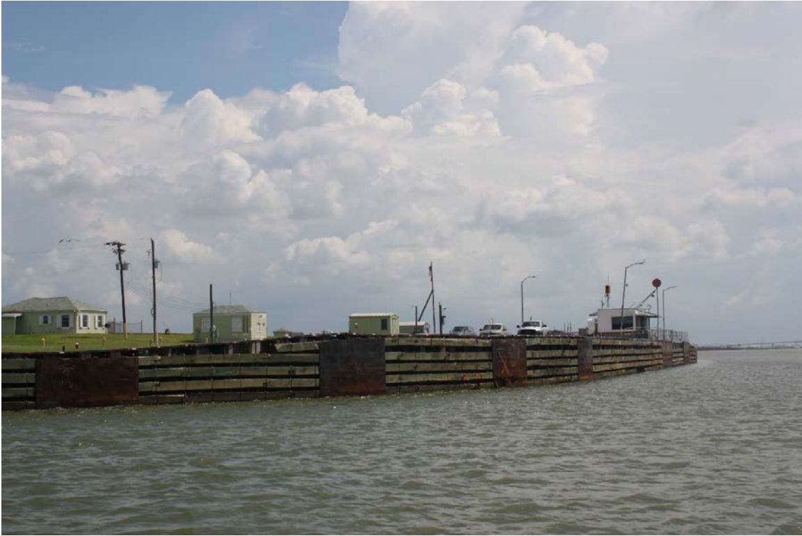
View of north guardwall, facing north
