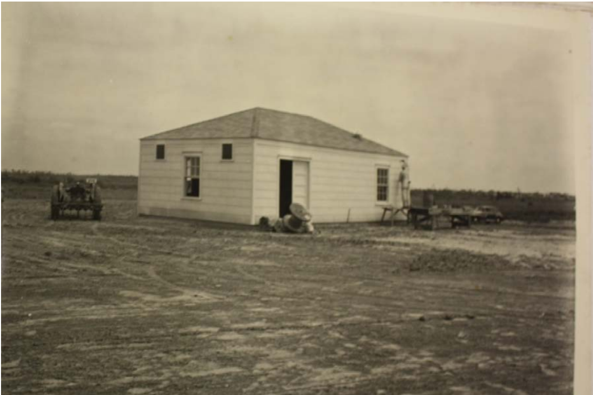
Photo dated 1944 showing power house, facing north
