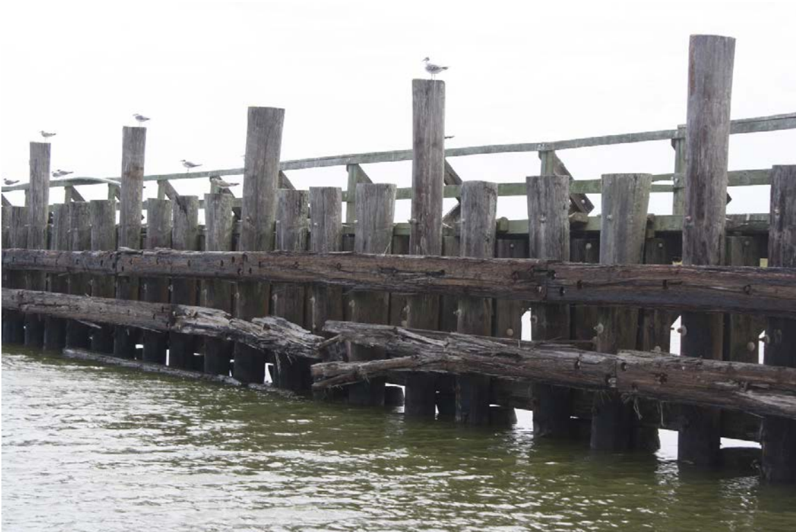
Representative photo showing damage to lock chamber timber guide wall, facing northwest
