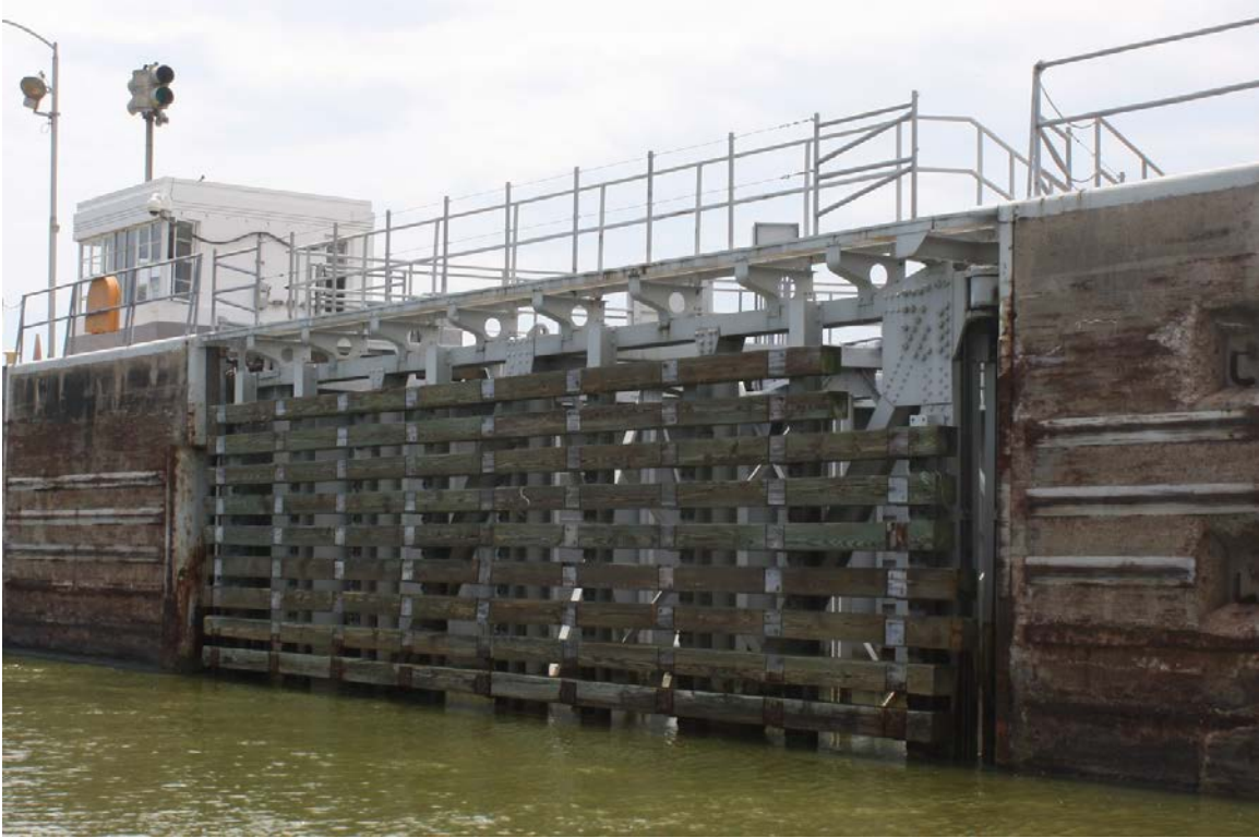
View of 1951 north lock gate, facing west
