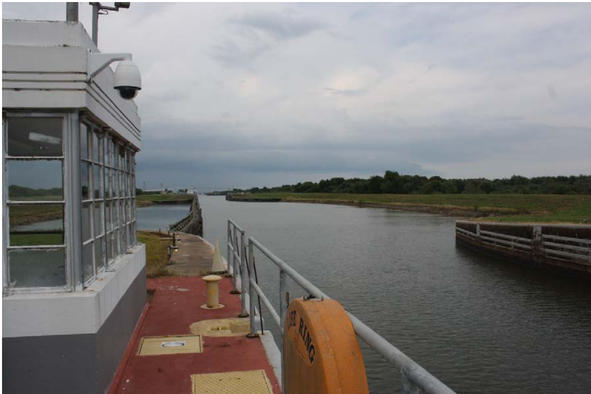
D20: View from 1951 control house toward south bank (historically devoid of structures aside from gates) and lock chamber, facing northeast
