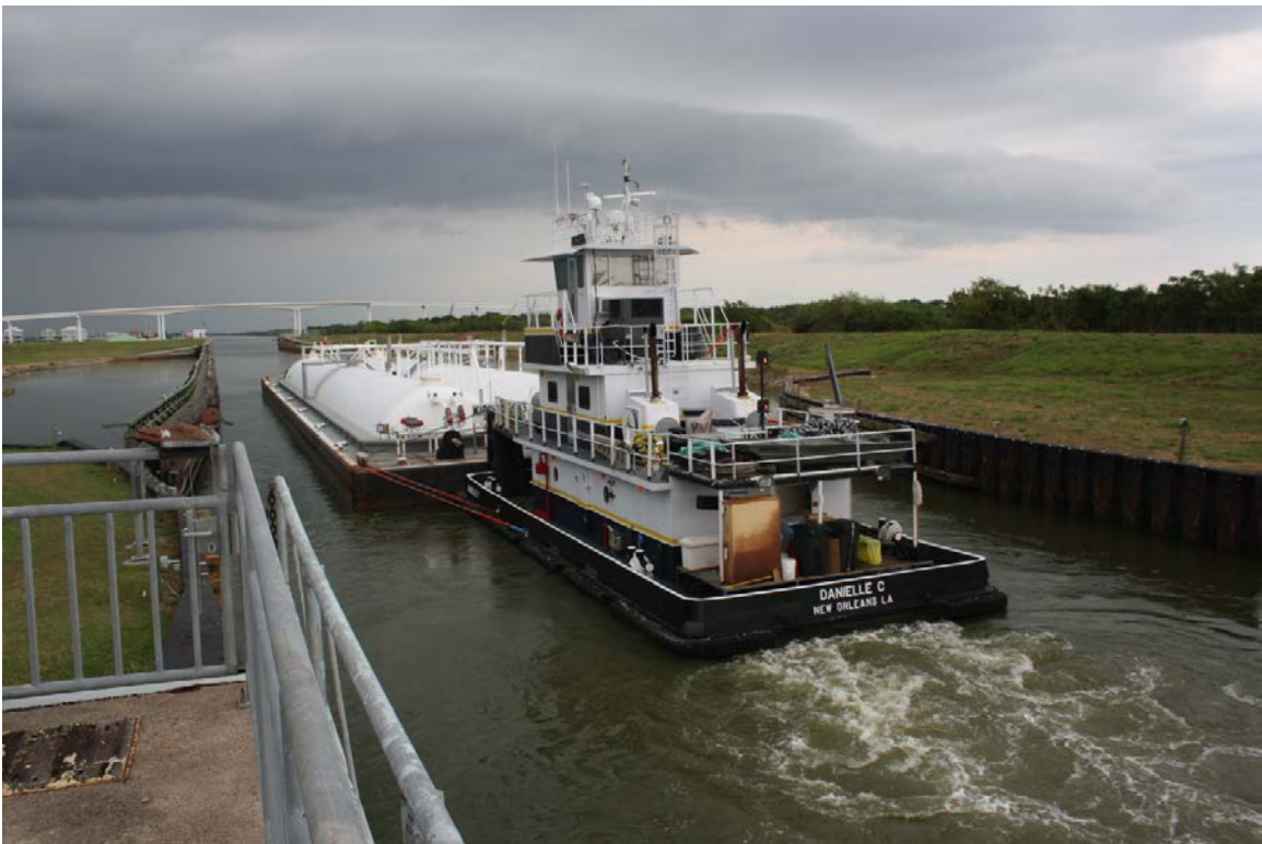
D36: View of barge traveling east through east locks and lock chamber, facing east
