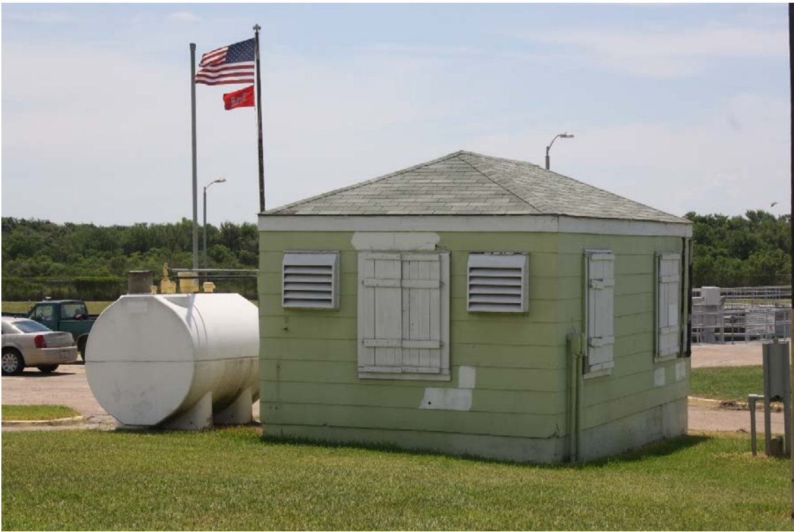
View of north elevation, facing southeast
