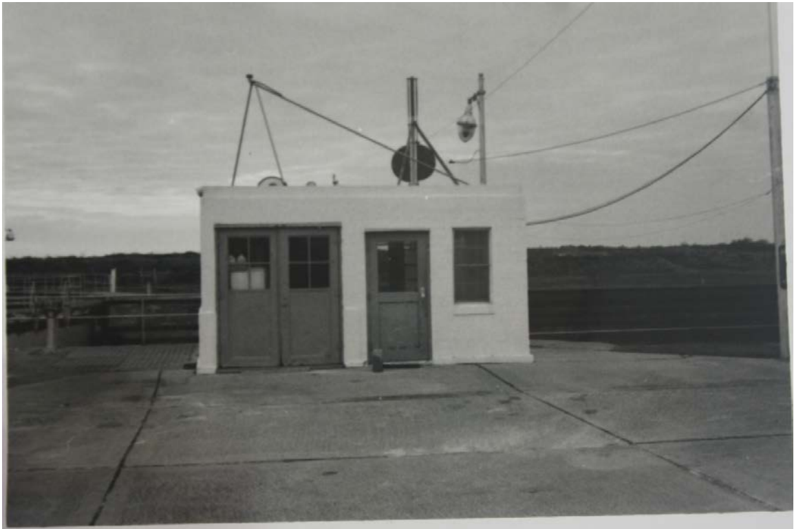
Photo from 1969 showing rear (north) elevation of control house, facing southeast. Image courtesy of USACE.
