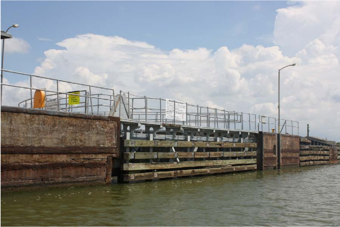
View of north gate, facing north
