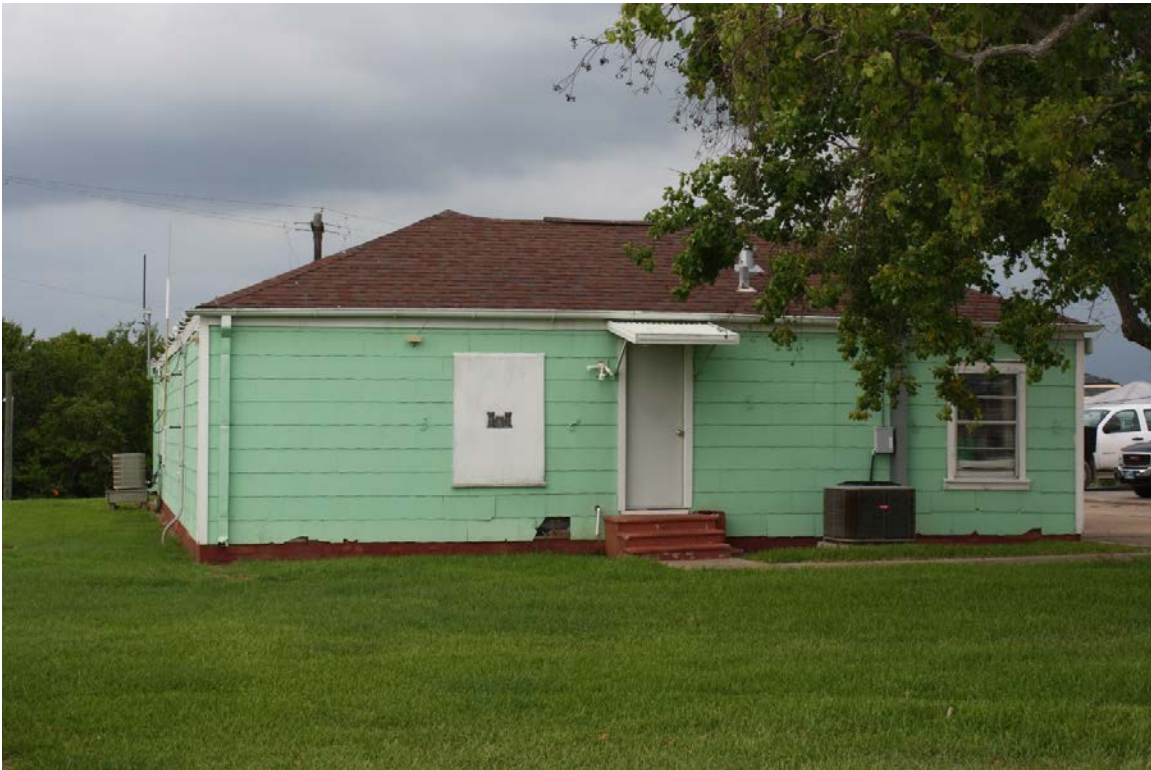
View of south elevation, facing north
