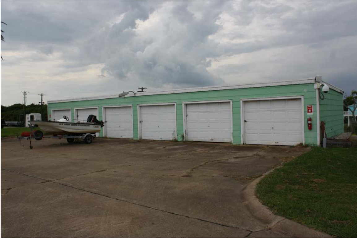
View of garage, facing west
