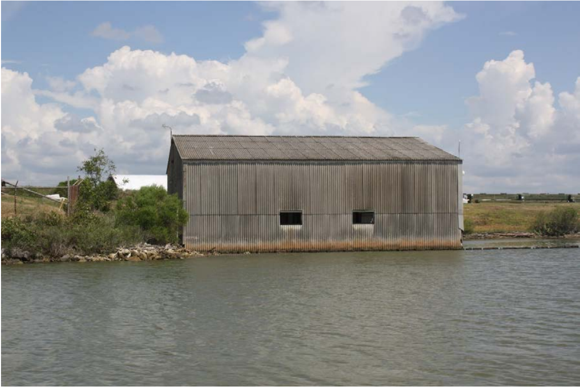
View of south elevation, facing northwest from the GIWW
