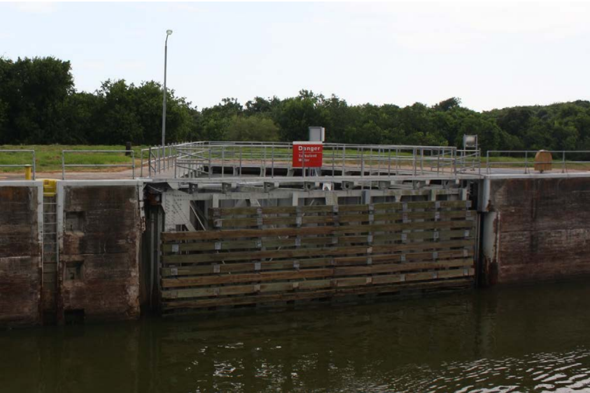
View of 1944 south lock gate, facing south
