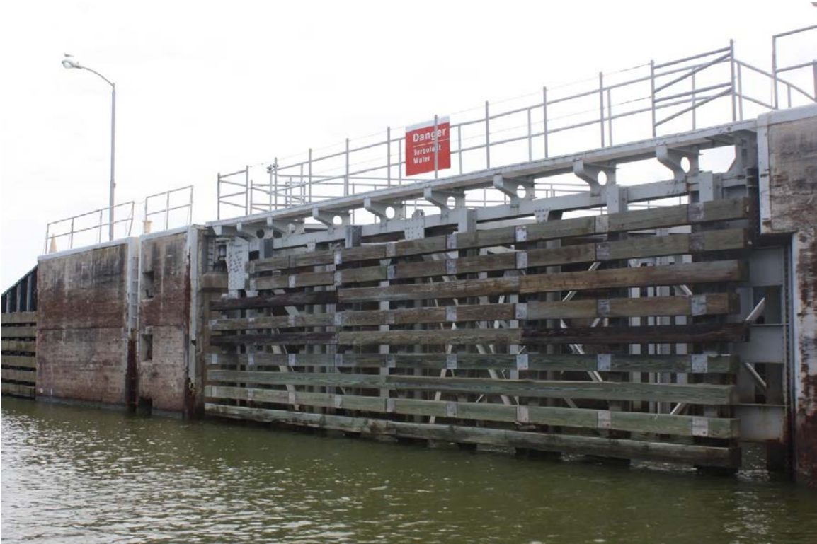
View of 1944 north lock gate closest to Colorado River, facing west
