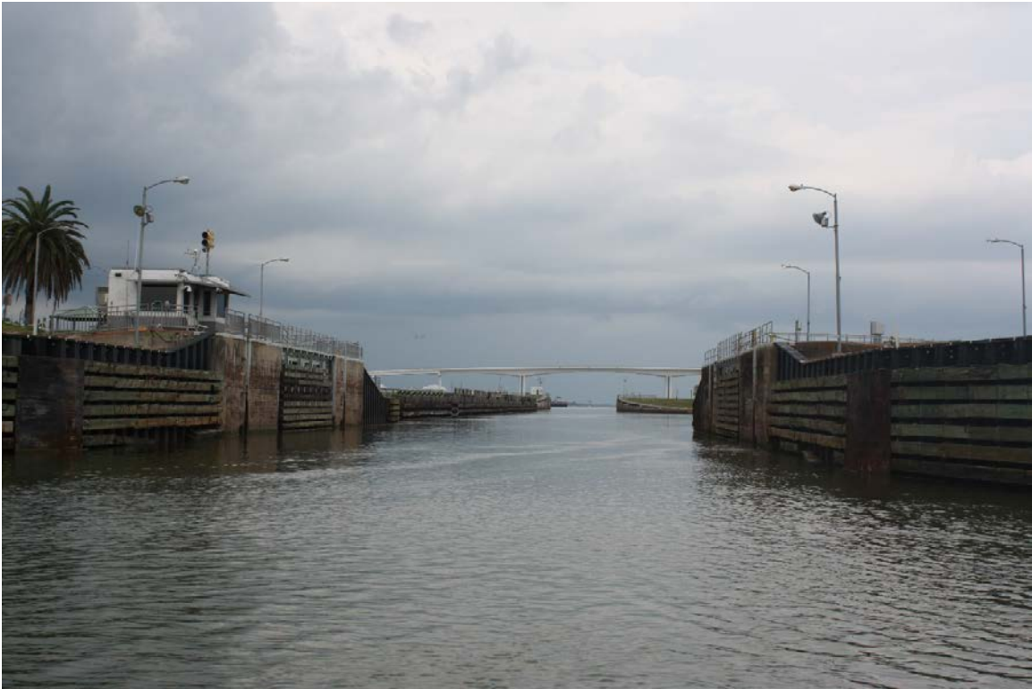
View of 1944 lock gates and guide walls, facing northeast
