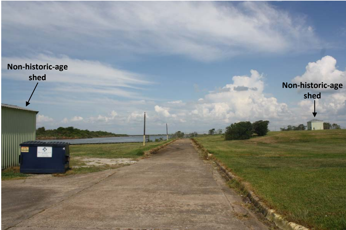
D7: View of west floodgate internal access road, facing southwest. Grassy area to the right used to have three residences.
