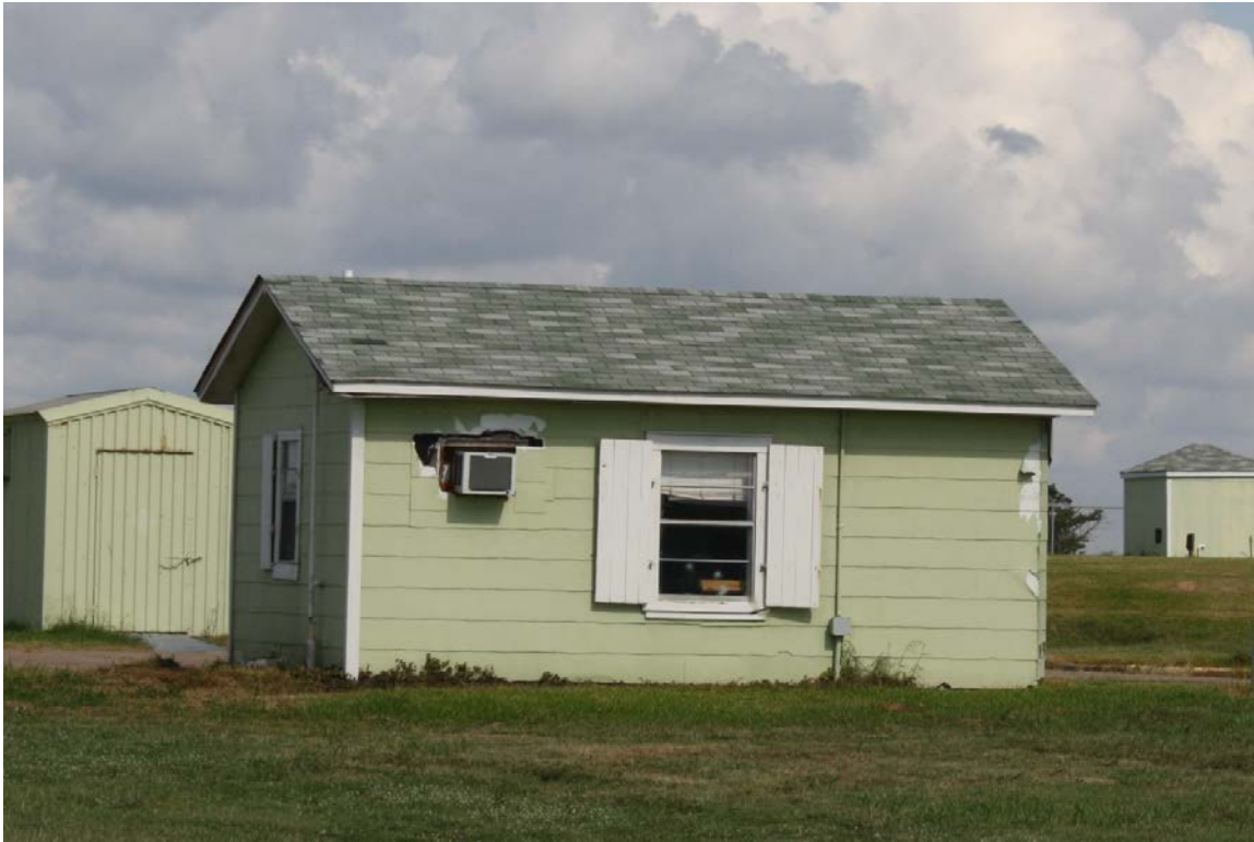
View of east elevation, facing northwest
