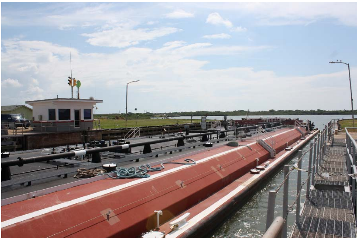
D8: View of barge traveling east through west floodgate, facing northeast
