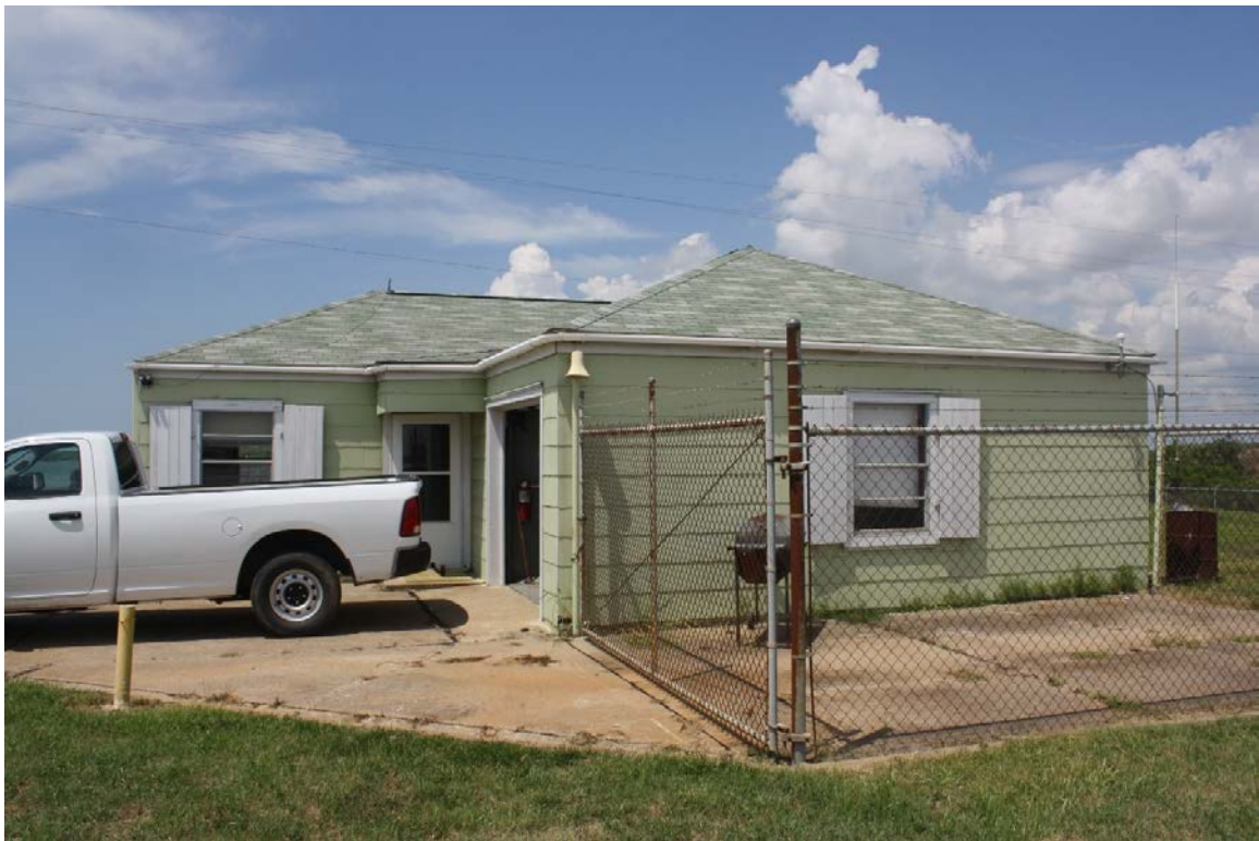
View of east elevation, facing southwest
