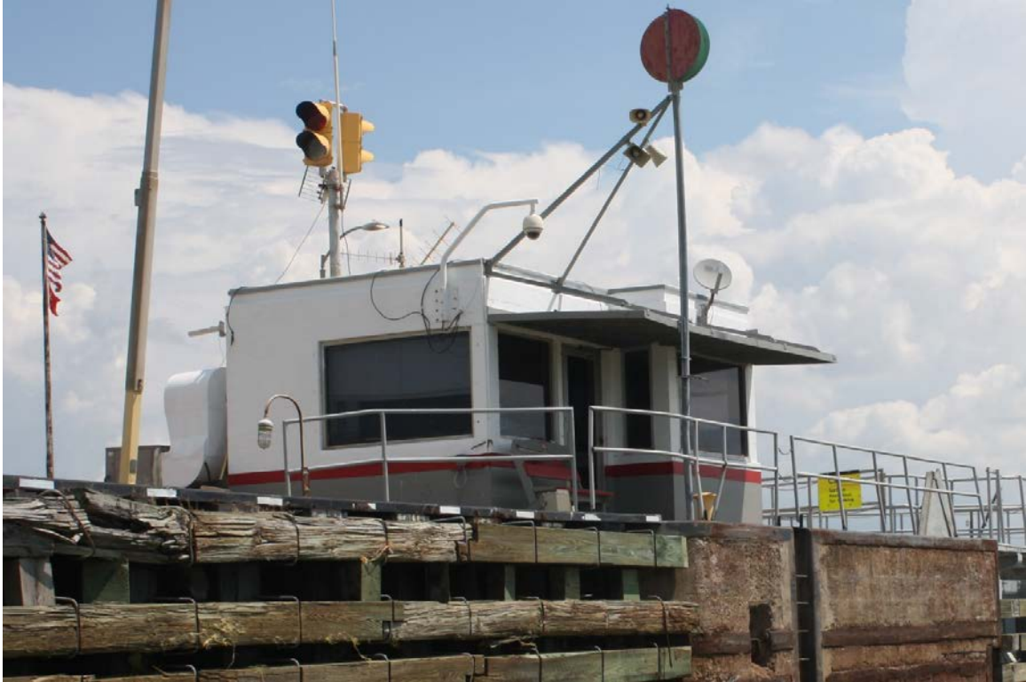
Oblique view, facing northeast
